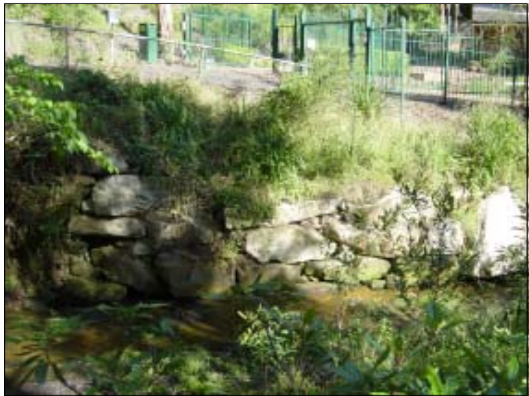
PHOTO 3: EXAMPLE OF BANK REVETMENT
