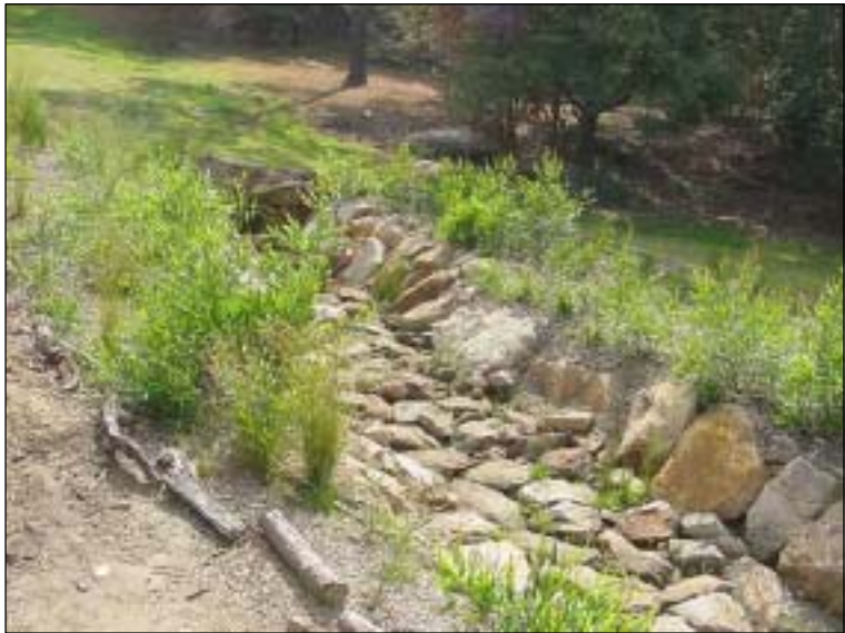
PHOTO 1: EXAMPLE OF RIFFLE STRUCTURES
