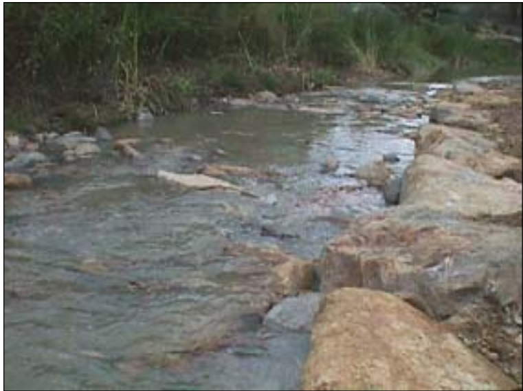
PHOTO 1: EXAMPLE OF RIFFLE STRUCTURES
