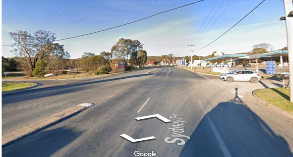
Figure 4 - Intersection Sydney Road and Common Street (Google Maps)
