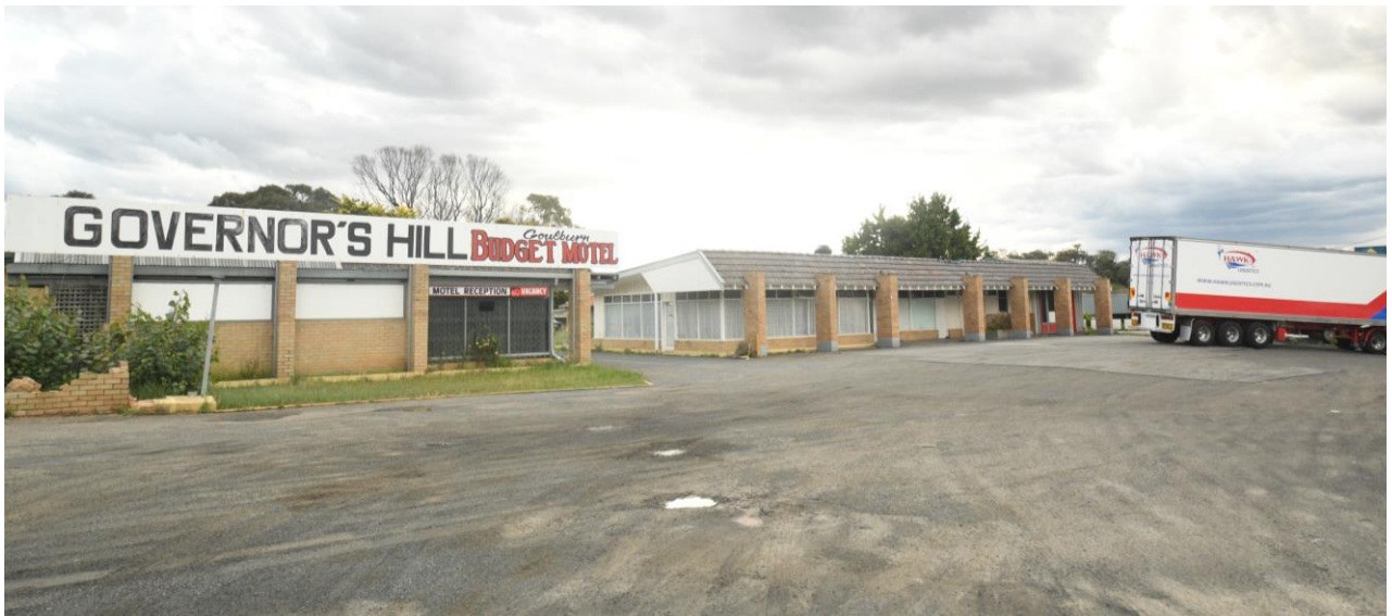
Figure 1-3 Existing hotel as viewed from Sydney Road
