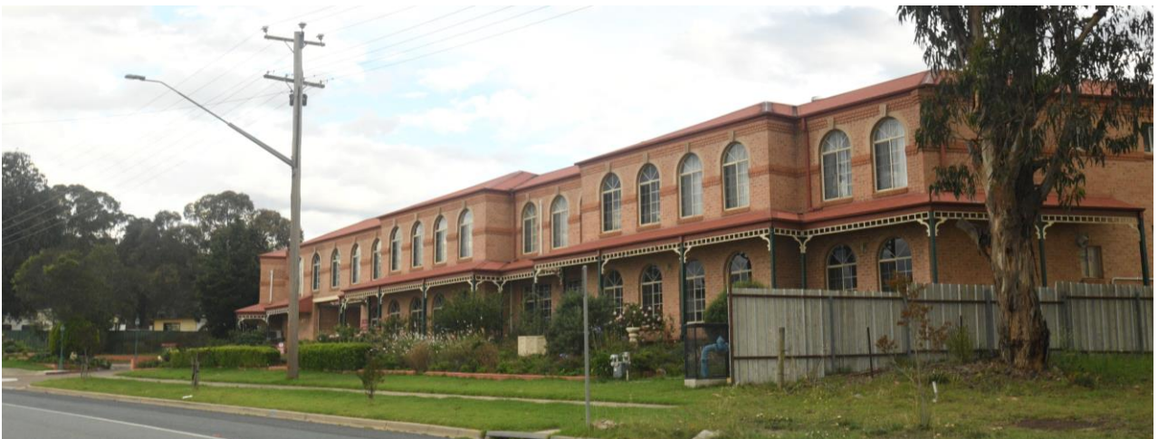
Figure 1-9 Existing hotel to the east of the subject site
