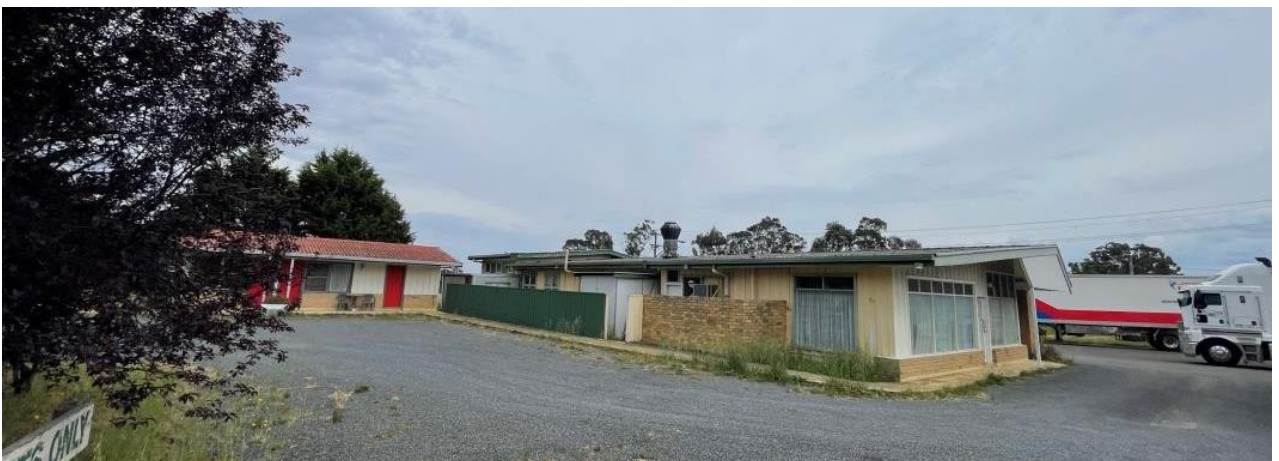
Figure 1-6 Site as seen from the internal carpark (Source: Neo Consulting)
