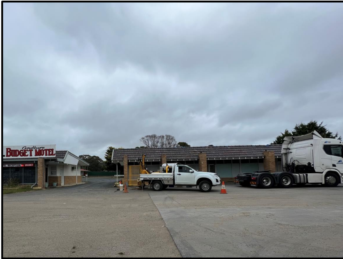
Figure 9. Building structure within the southern portion of the site.
