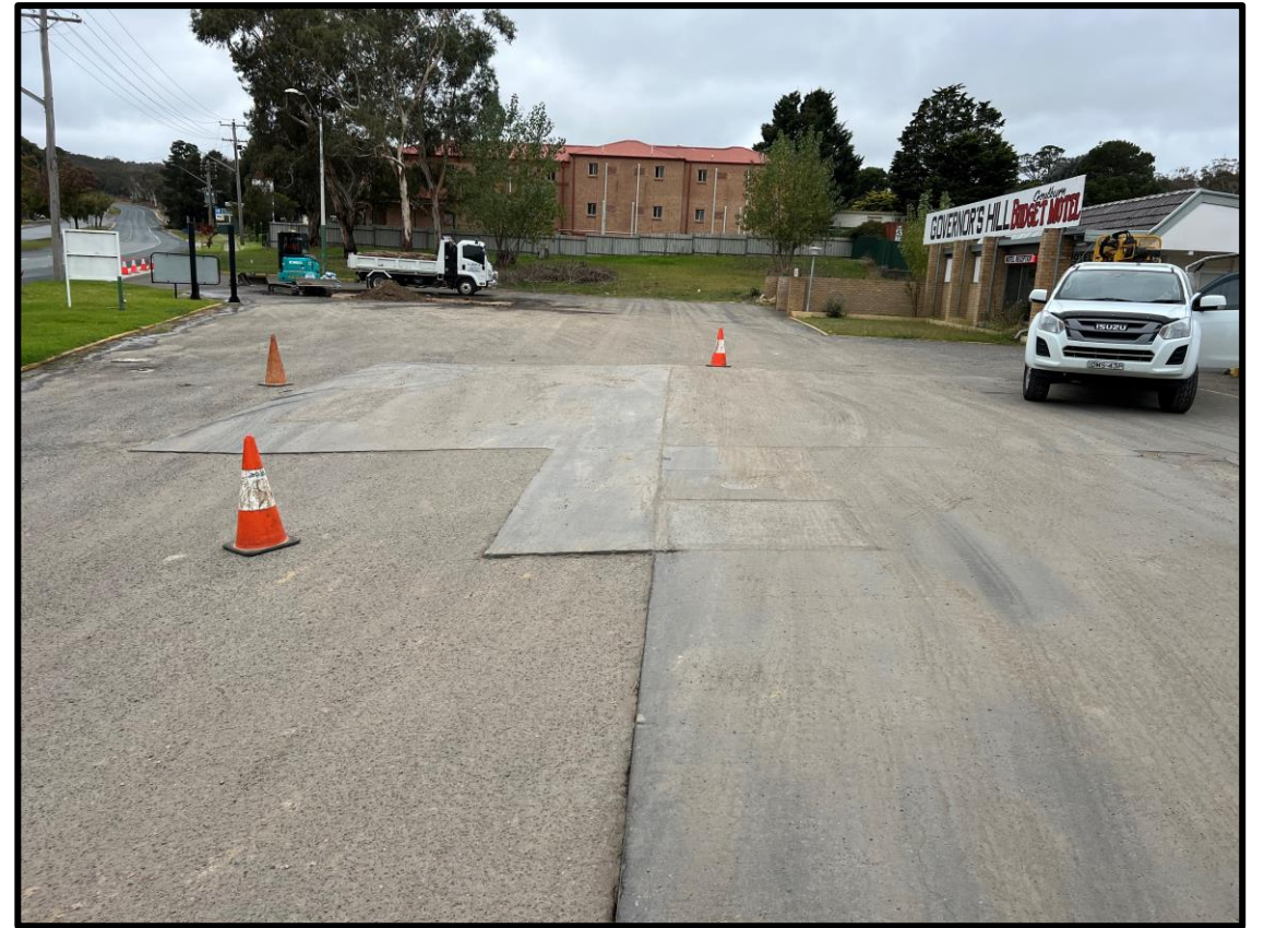
Figure 10. Eastern portion of the site and the concrete groundcover.
