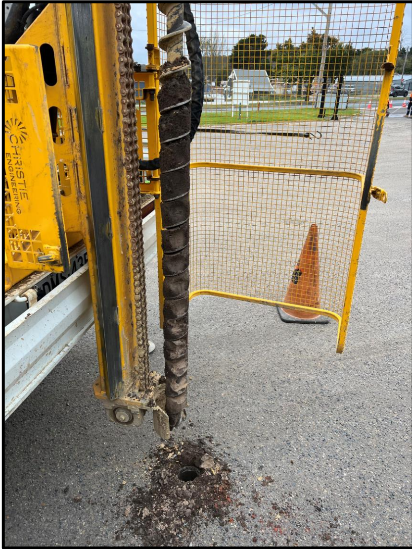
Figure 13. Drilling of BH1.
