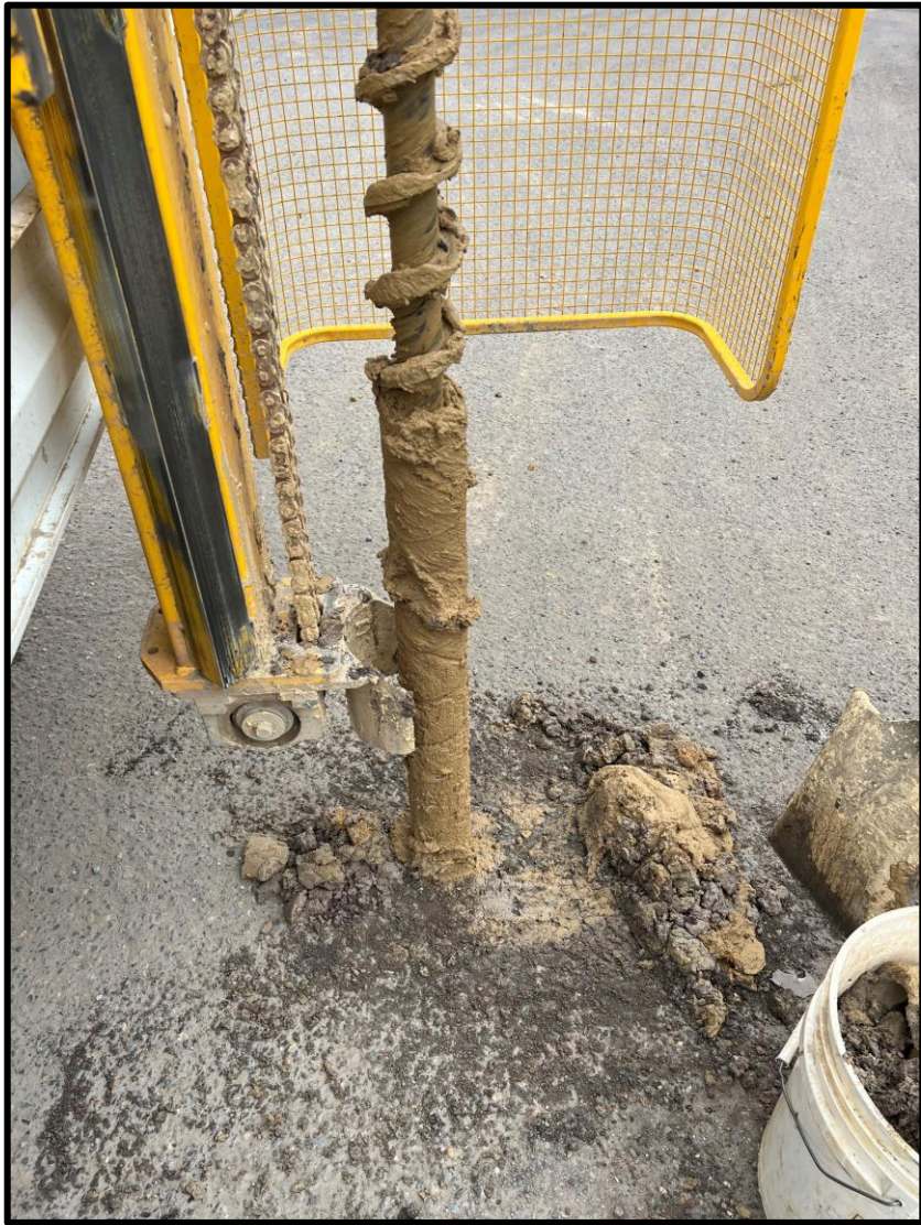
Figure 15. Drilling of BH5/MW1.
