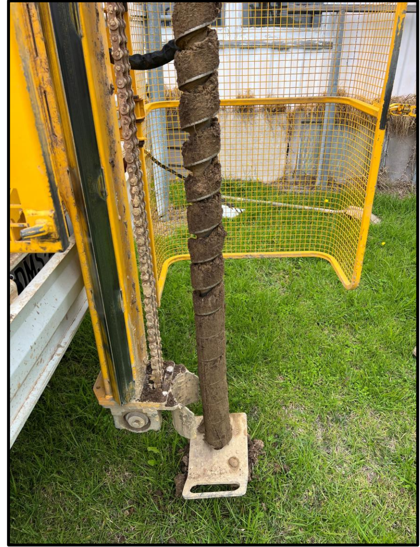
Figure 14. Drilling of BH8.
