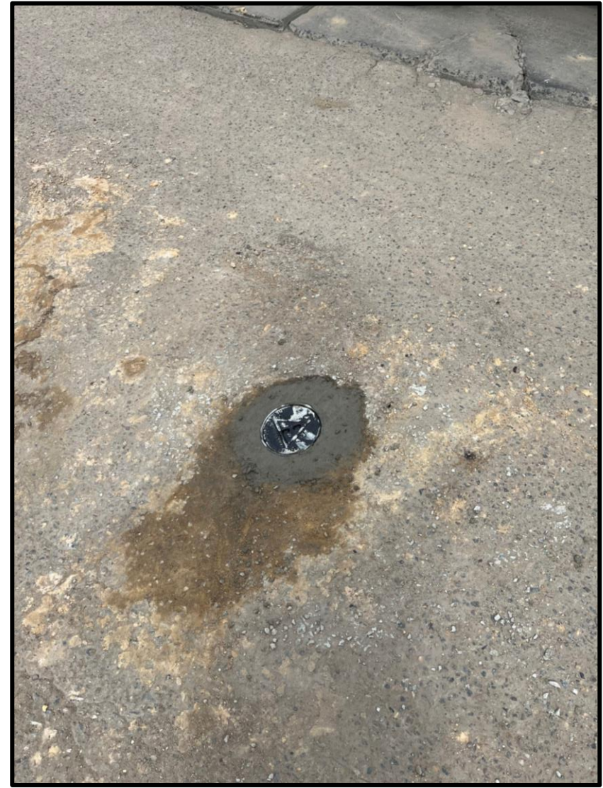
Figure 16. Installation of MW1.
