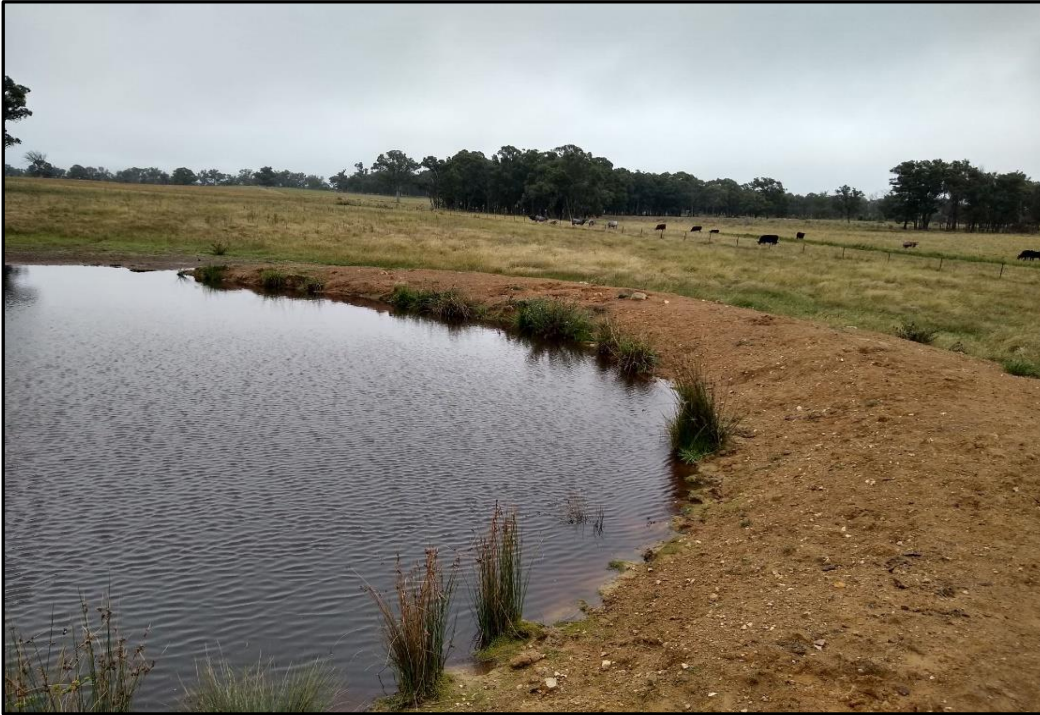
Photo 5: View of the dam in the western portion of the site
