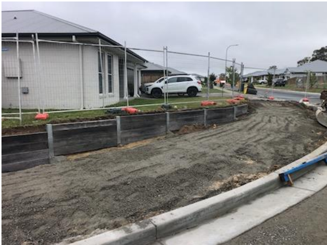
Figure 3: Typical retaining wall – sleeper wall
