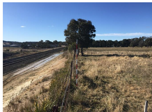
Plate 9: Northern boundary fence line adjacent to the railway easement (East)
