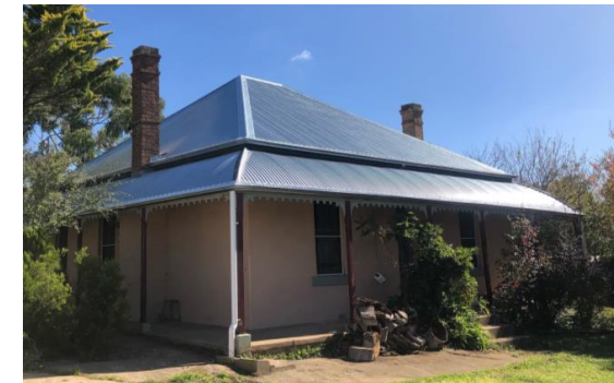
5 Kadwell Street, Goulburn Roof restoration
