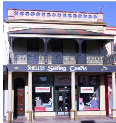
115 Auburn Street, Goulburn Paint restoration
