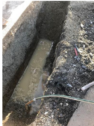
Water Main Combermere Street 2022-23
