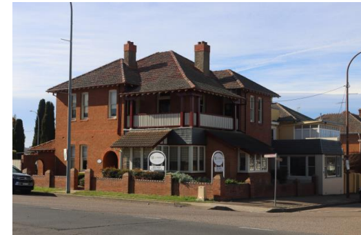
33-35 Montague Street, Goulburn Paint restoration
