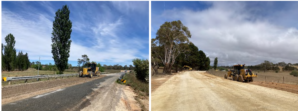
Windellama Road Stage 5 – Gravel overlay in progress
