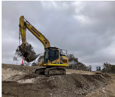
Reader Road – Bulk Earthworks
