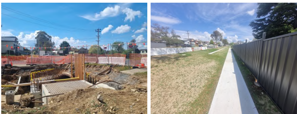
Faithfull Street - Stormwater works
