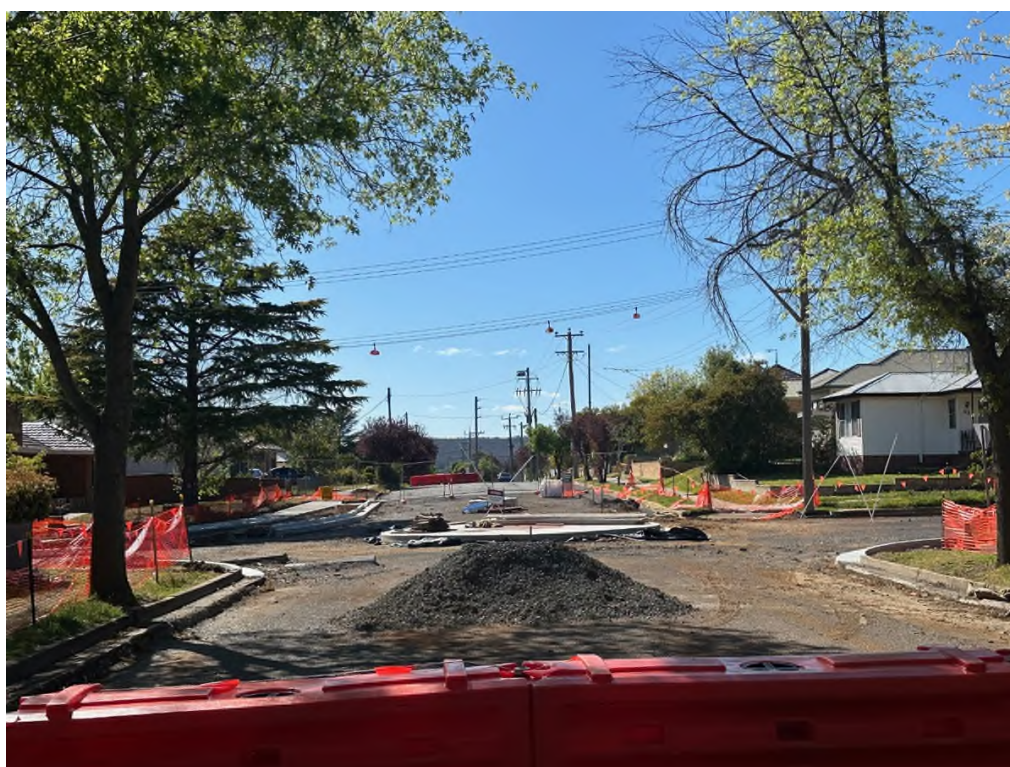
Kinghorne Street worksite
