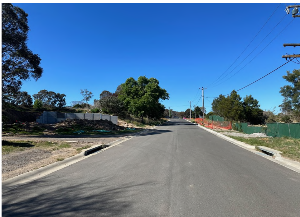
Common Street – Substation retaining wall
