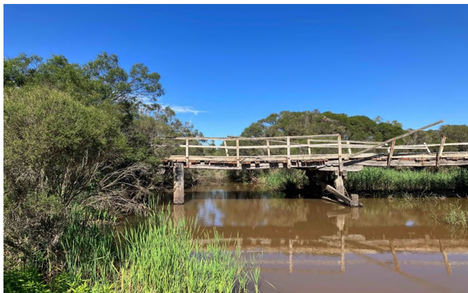
Mayfield Road Bridge – Closed with diversions in place.
