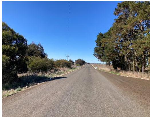
Painters lane Intersection – Bitumen Sealed
