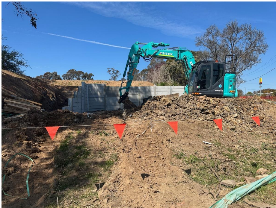
Common Street – Work in progress
