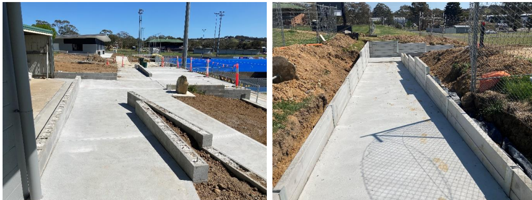
Hockey Centre Amenities Block – Current progress
