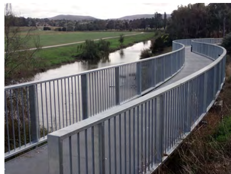
Above: An elevated section of the RiverWalk along the Wollondilly River
