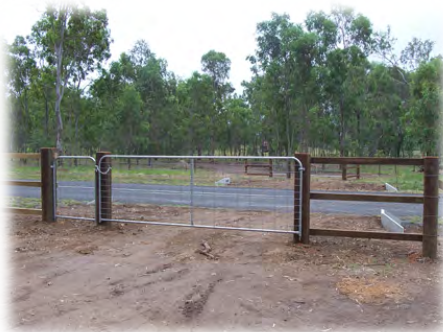
Self-closing trail user access gate and locked management access gate at a road crossing on the Brisbane Valley Rail Trail.
