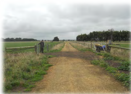
Cattle crossing gates, as used on the Port Fairy Warrnambool Rail Trail in Victoria, enable adjoining farmers, and their cattle/sheep, to cross the trail whenever necessary – thereby not hindering farming practices. Gates are closed across the trail and side gates on side boundaries opened to allow stock to cross when required. This spectacle - when it occurs - is of considerable interest to trail users.
