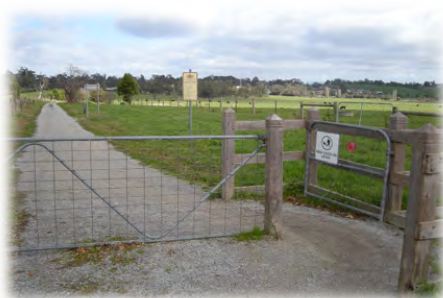
The gating system at road crossings used on the Lilydale Warburton Rail Trail in Victoria makes it difficult for unauthorised users (such as motor bikes and 4WD vehicles) to gain access to the rail trail.
