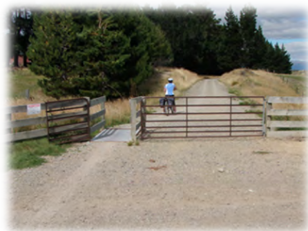
Grids are commonly used on rail trails at fence lines and property boundaries to prevent stock from escaping, but still allowing the passage of cyclists and walkers. This example is from the Otago Central Rail Trail in New Zealand. Similar examples can be found on the High Country Rail Trail in Northern Victoria.
