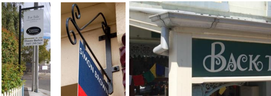
Figure 3.5: Good Examples of signage on heritage buildings and in heritage areas
