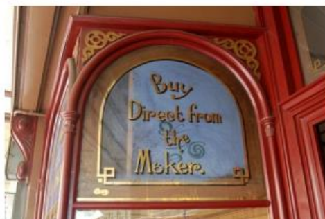
Figure 3.13: Shopfront examples - Style elements include retention of original details such as ceramic tiles, symmetrical layout, ornamental timber joinery, decorative signage on glazing, retention of original shopfront framing.
