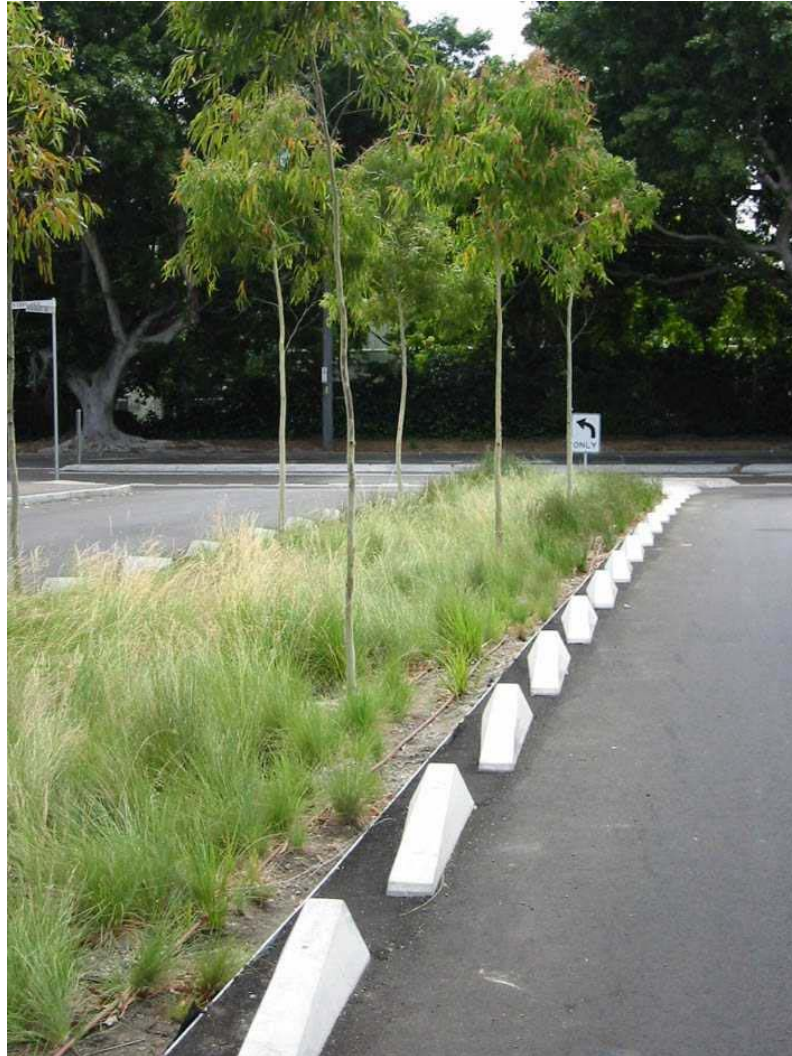
Plate 3: Bioretention Trenches at Victoria Park, Sydney
