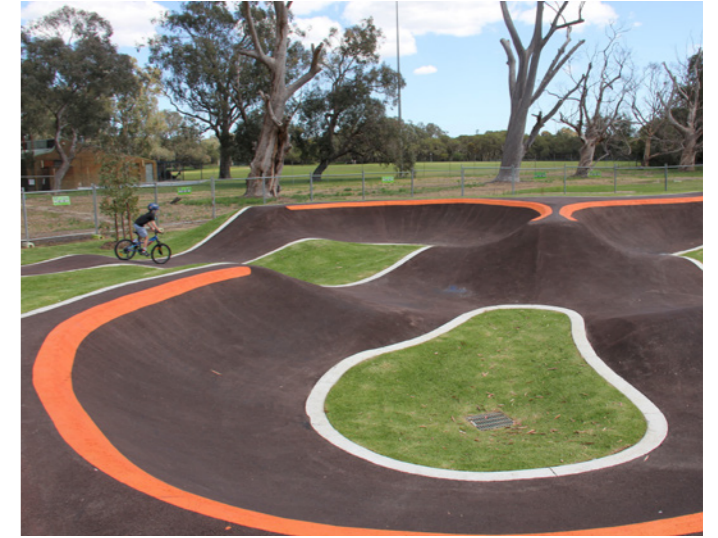
Intermediate loop and features. 800mm high berms, 400-600mm high features
