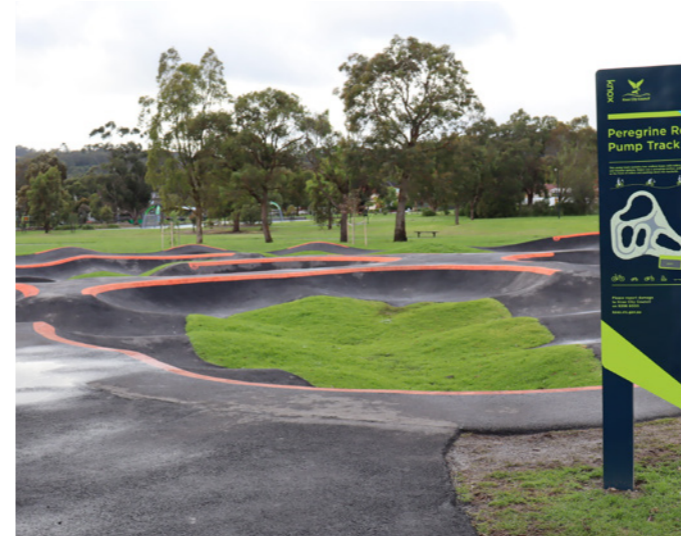
Beginner loop and features. 800mm high berms, 400mm high rollers
