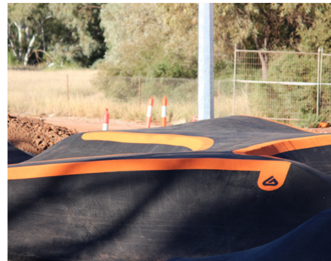
Back to back berm
