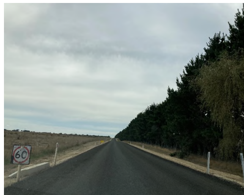
Bitumen Sealing Works – Stage 4
