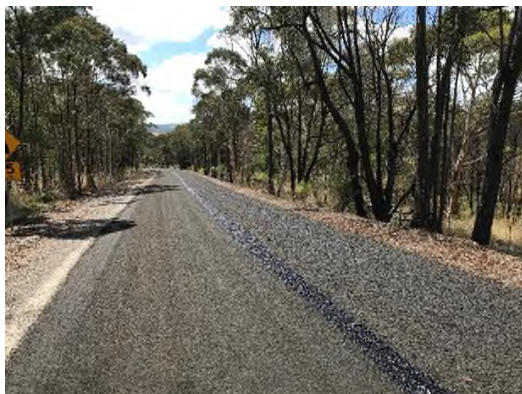
Bitumen Sealing- Stage 3 Works
