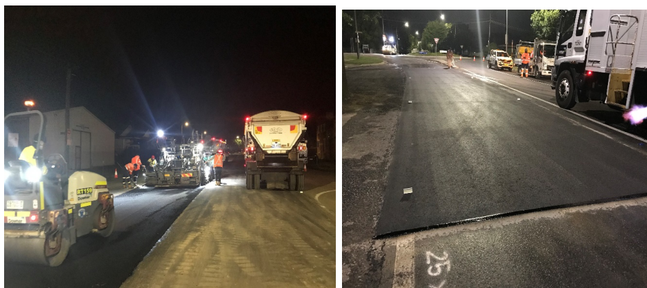
Urban Asphalt Works – Bradley Street & Victoria Street
