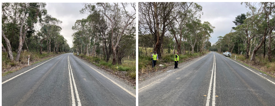
Pavement Works – Highland Way Road
