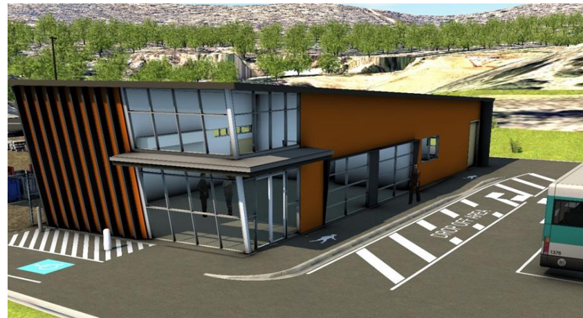
A new Re-Use Hub (tip shop) is under construction at Goulburn Waste Management Centre.
