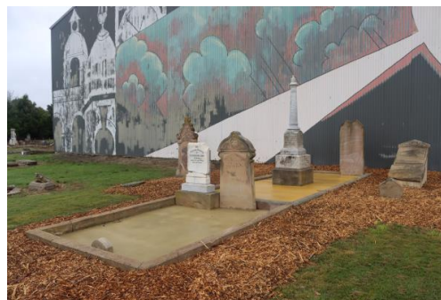
Conservation of Graves at Mortis Street Cemetery
