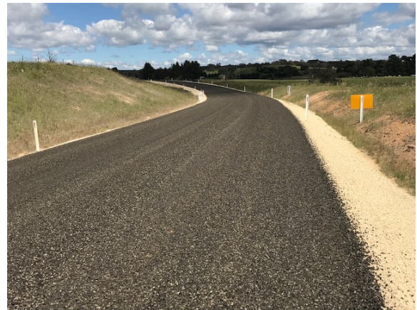
Windellama Road Construction Sealing
