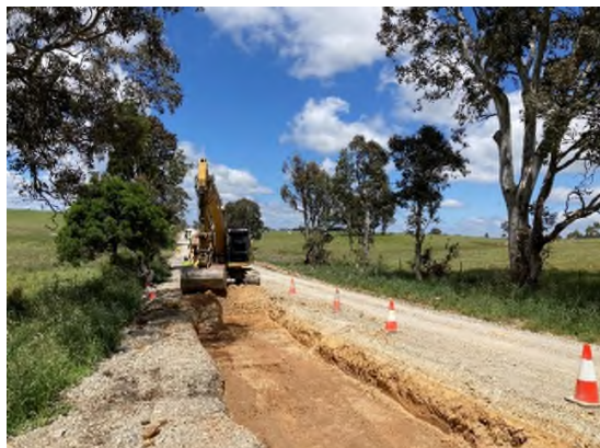
Windellama Road Stage 2 Pavement Works
