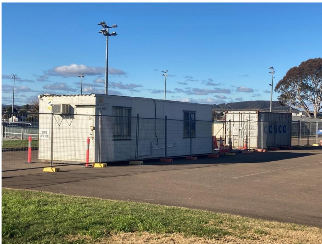
Hockey Centre – Site Establishment
