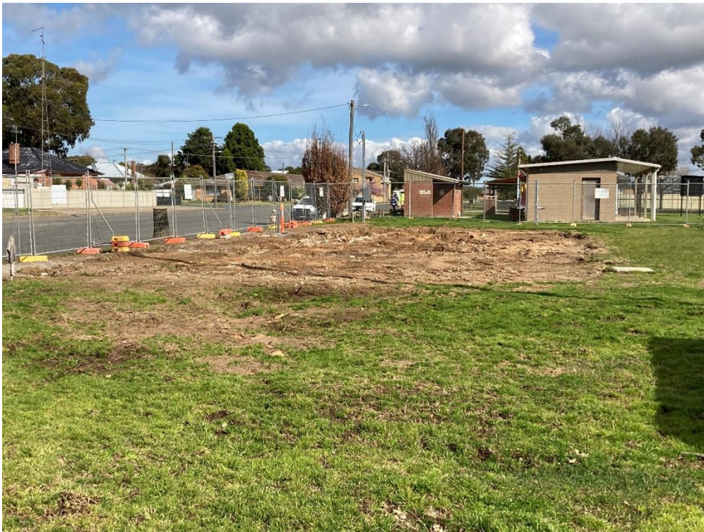
North Park – Demolition Complete
