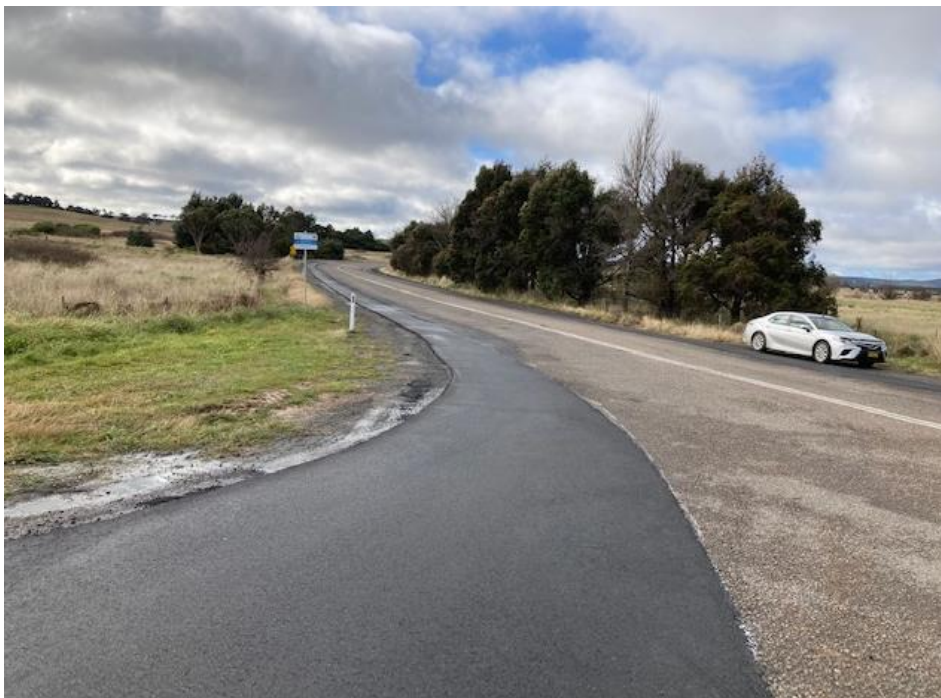
Asphalt edge widening within Stage 1
