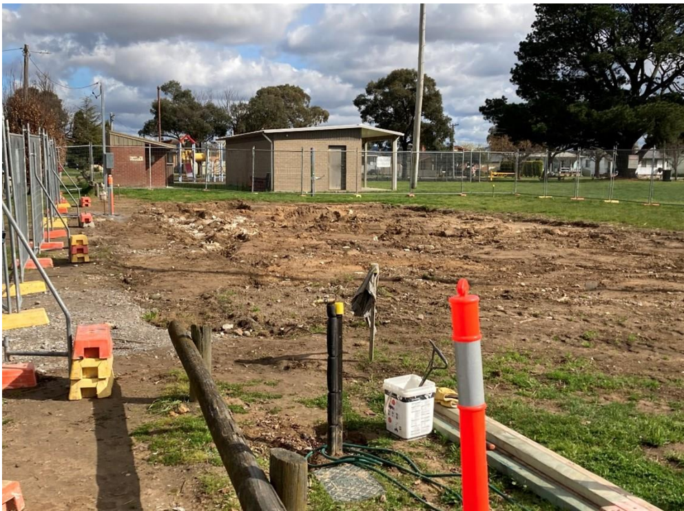
North Park – Demolition Complete
