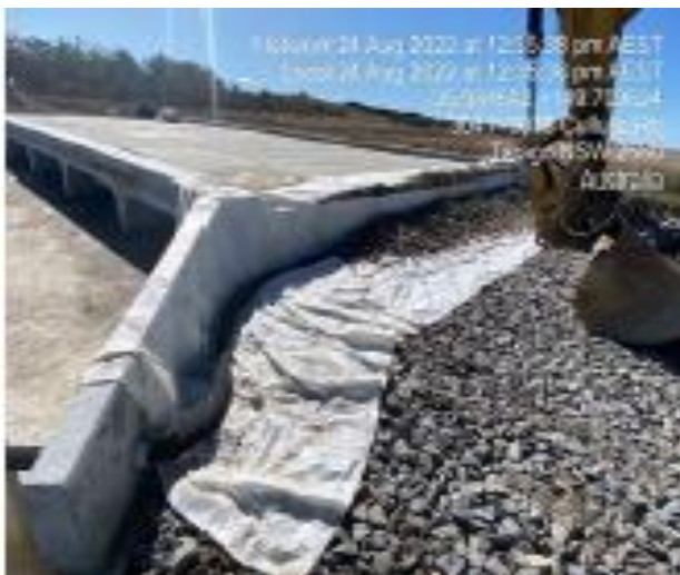
Progress at Cullulla Causeway Replacement Project
