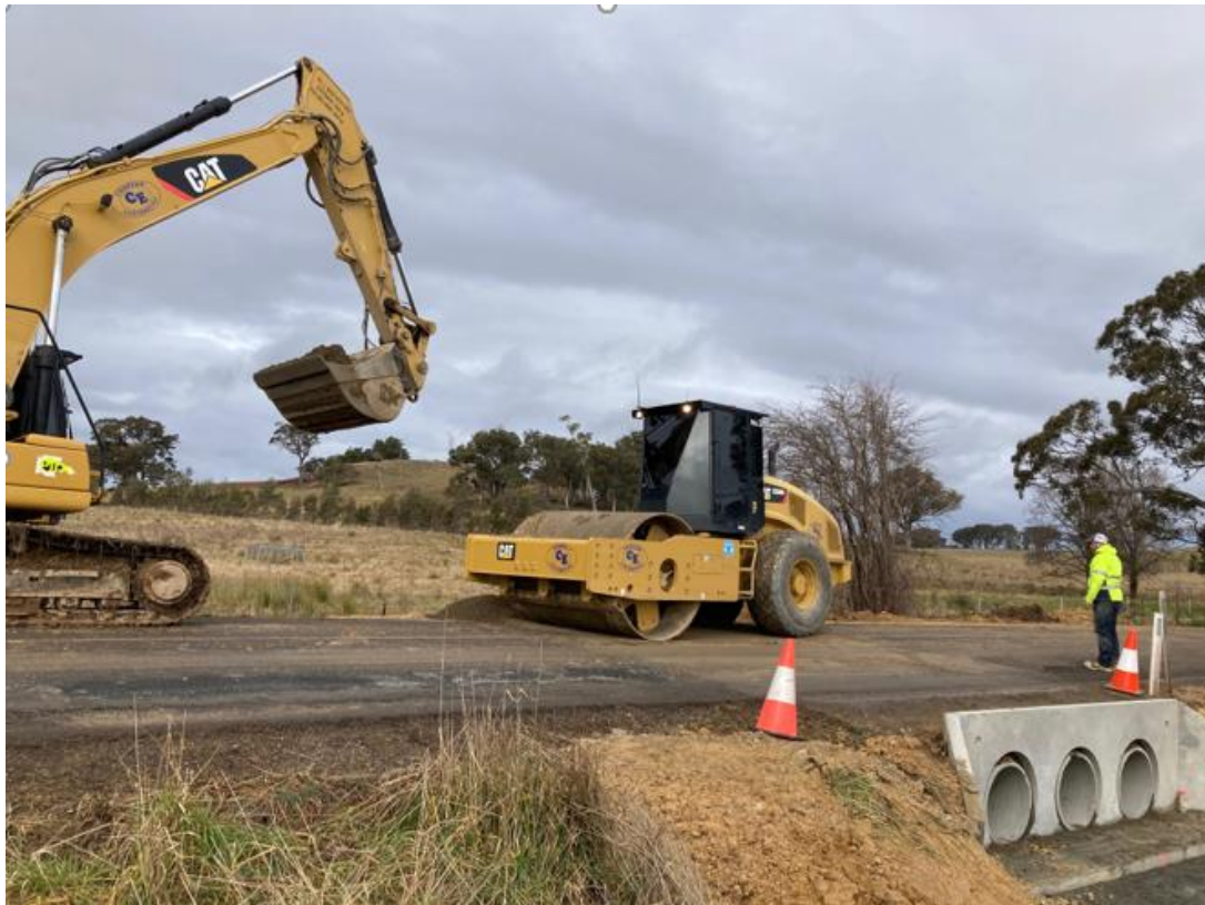
Stage 2 trench compaction
