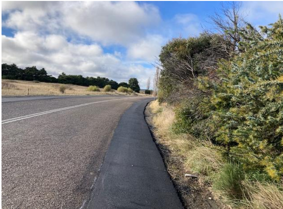
Asphalt edge widening within Stage 1
