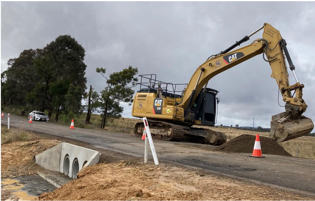
Stormwater extension within Stage 2
