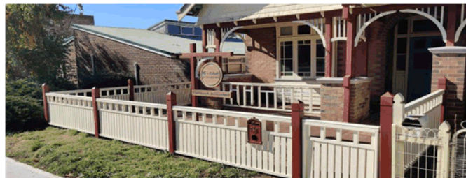
New front fence installed at 177 Bourke Street with the help of Heritage Grants
