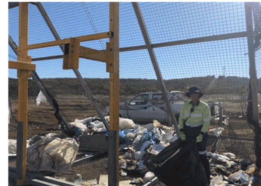
Litter nets now surround the Goulburn’s landfill, helping to reduce wind blown litter
