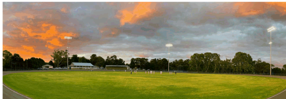
New lightining installed at Seiffert Oval
