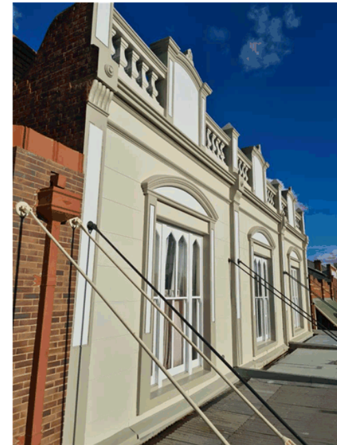
131 Auburn Street – Paint façade. This project completed the painting of the last one of a group of three attached shops in Auburn Street. All three properties received CBD Grant Funding
