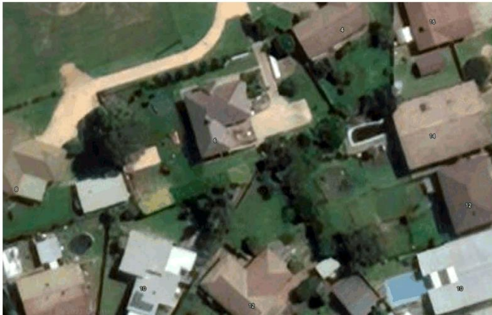
Aerial view of Lot 151 showing the size of Lot 151, and the large boundary setbacks from the adjoining lots and dwellings.
