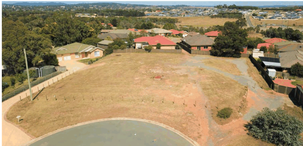
Photo showing the single storey gable and hipped roof construction of the neighbouring houses.
