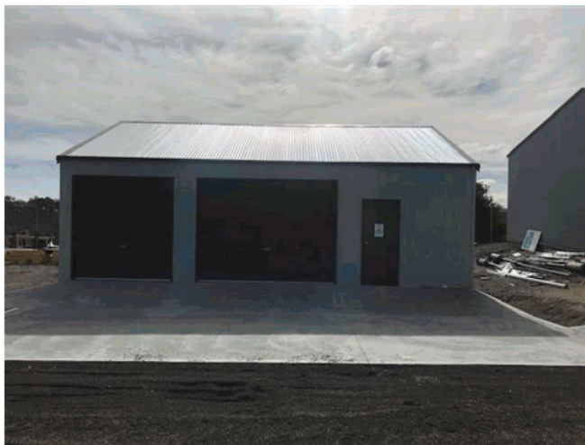
Hetherington Street Depot – Weeds Shed
