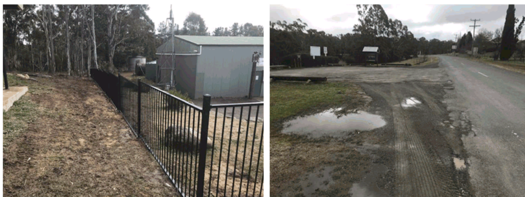
Fire Shed Fence and Bungonia Park Car Park
