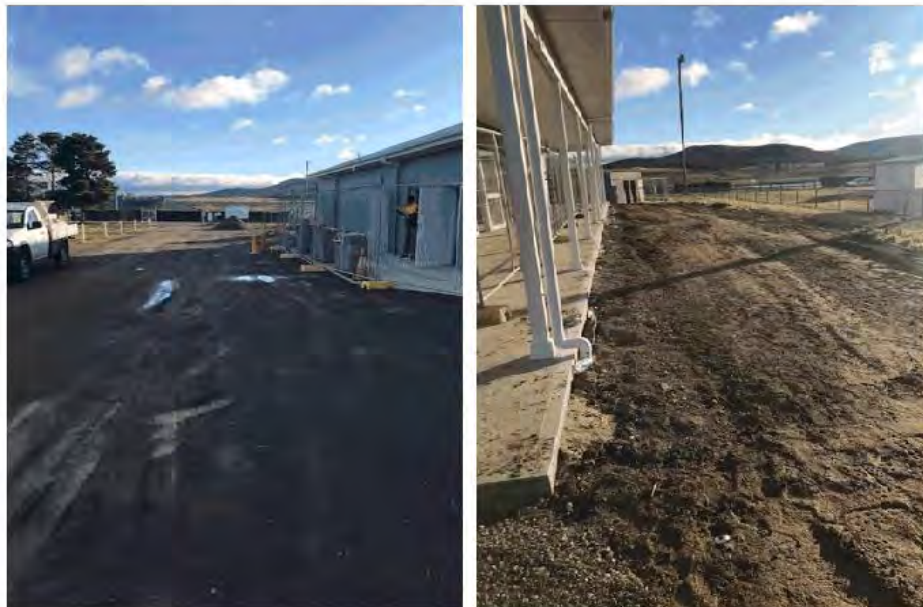
Cookbundoon Pavilion – backfilling of eastern and western side
