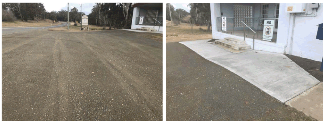
Community Hall car park (prior to sealing) and section of disabled ramp
