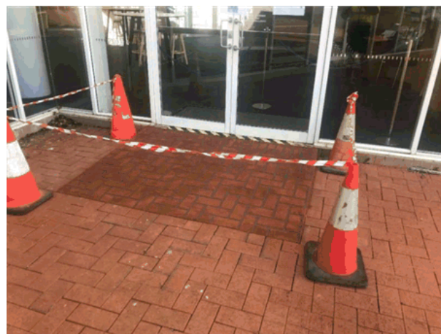
Chisholm Court All Access Ramp
