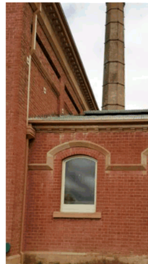
Masonry –GHW Pumphouse
