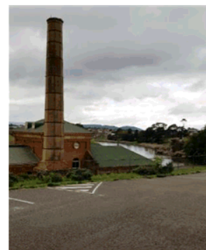
GHW Pumphouse and car park
