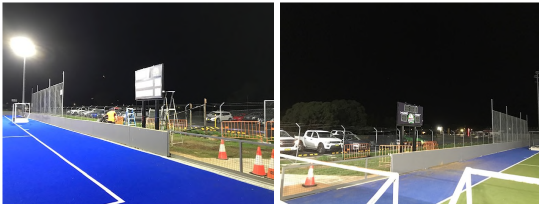
Goulburn Hockey Centre – New Scoreboards Installation
