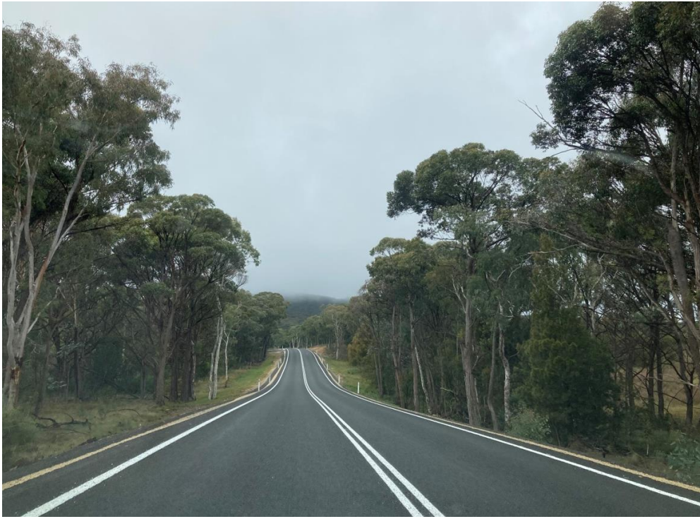
Bitumen seal and line marking within Stage 3
