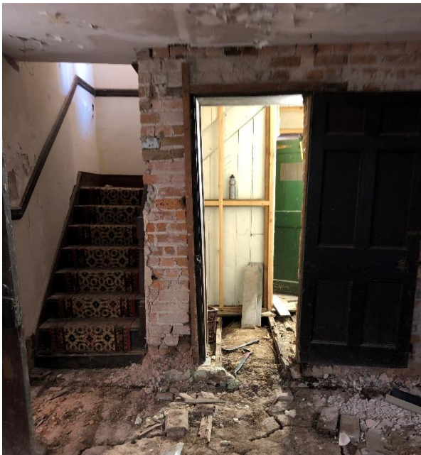
Villa – stairs during sub-floor works. Note the bricks on clay, and the lack of sub-floor clearance, contributing to rising damp issues.
