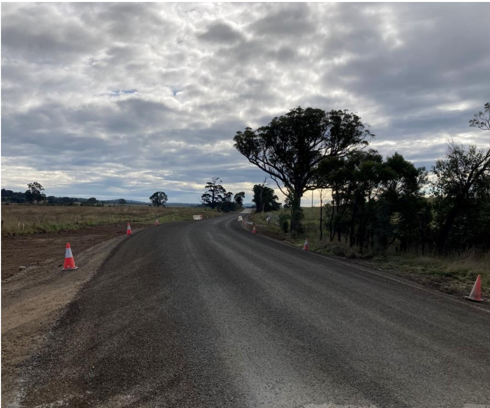
Bitumen sealing Stage 2
