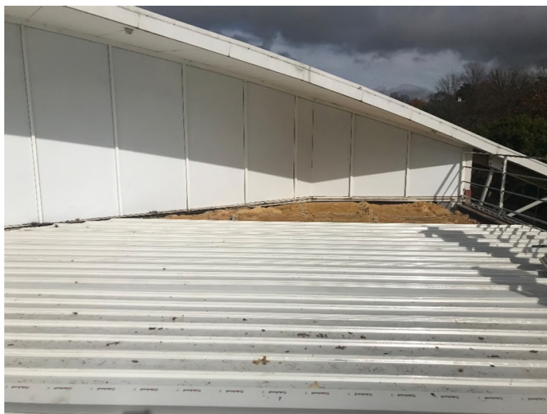
New roofing over foyer
