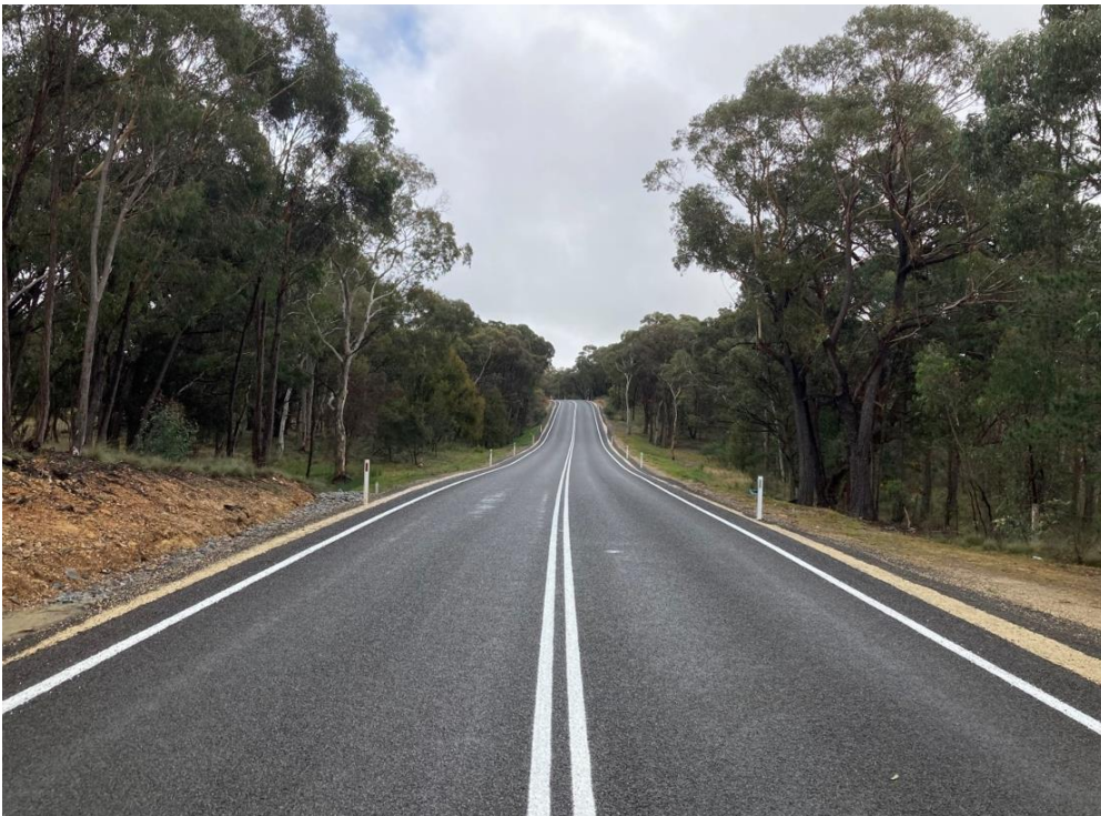
Bitumen seal and line marking within Stage 3
