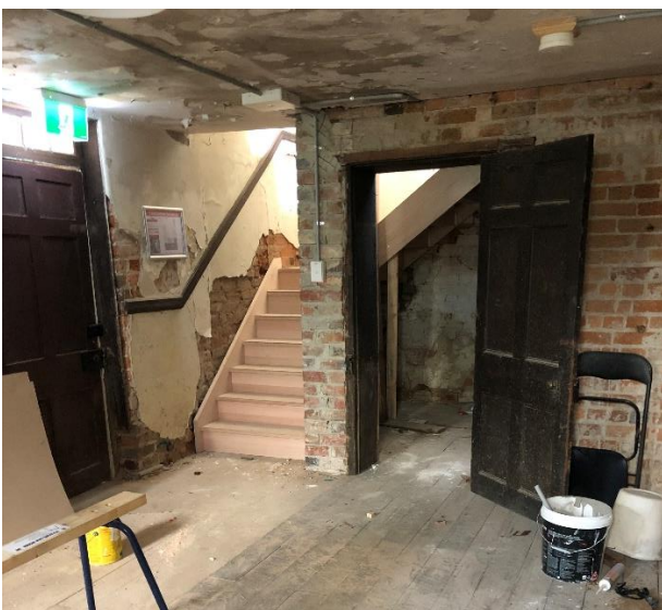
Villa – New compliant and structurally sound stairs in the process of being installed. Note re-build of wall, floors to be completed in June.
