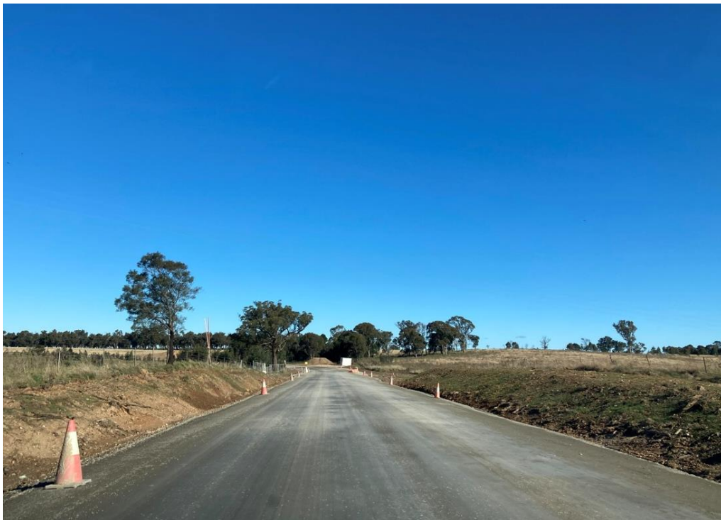
Base preparation Stage 2
