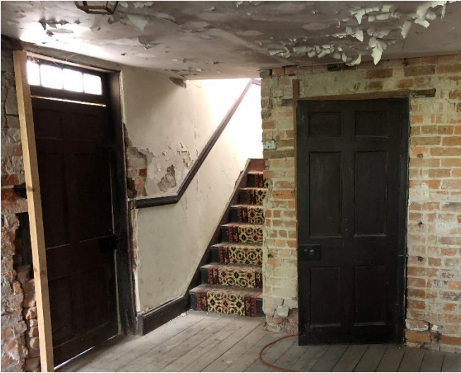
Villa – Original unsafe and non-compliant stairs (note this is before the sub-floor excavation works took place)
