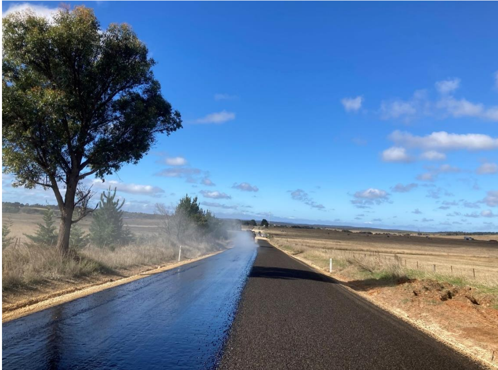
Bitumen sealing Stage 1
