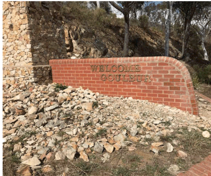
North Approach Entrance Wall
