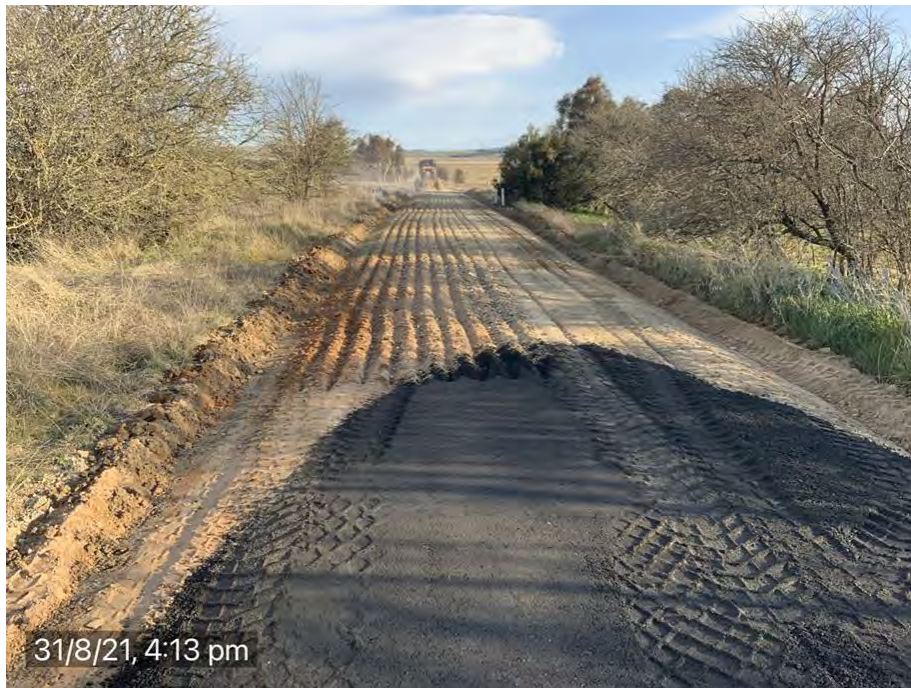
Parkesbourne Road gravel resheeting – Utilising reclaimed asphalt from TfNSW stockpile site
