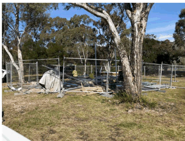
Tallong Amenities – Recommencement of Construction
