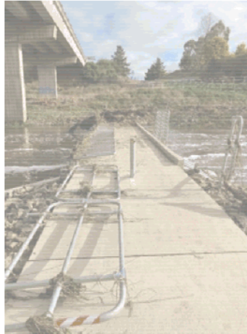
Wollondilly Walking Trail – Crookwell Road Bridge
