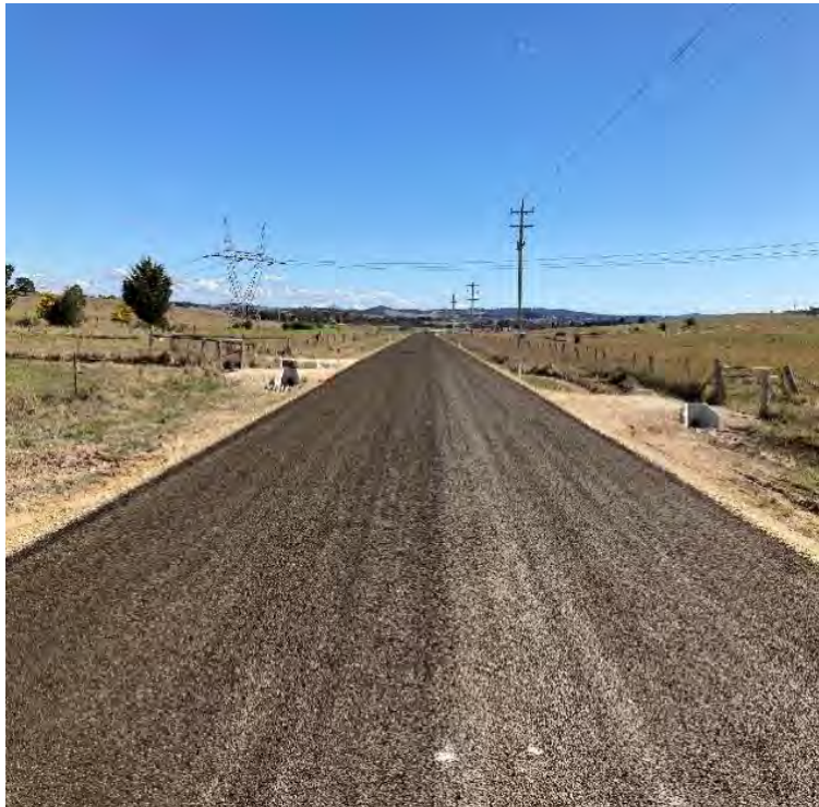
Stage 1 - 2.7km bitumen sealed
