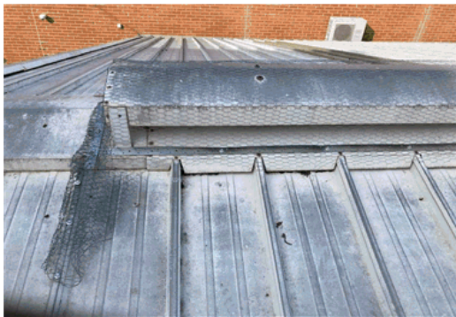
Poultry Pavilion Roof
