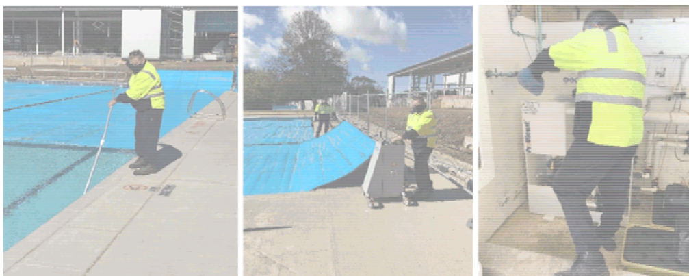
Staff repairing and carrying out maintenance for opening of outdoor pool
