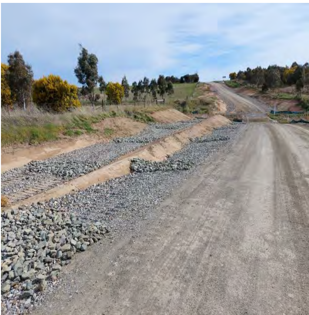
Drainage completed on Stage 2 of the project
