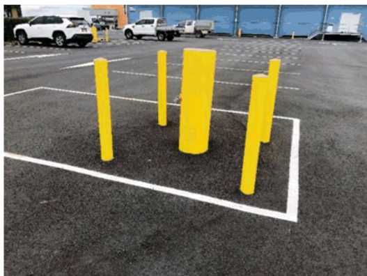
Car Park Bollards
