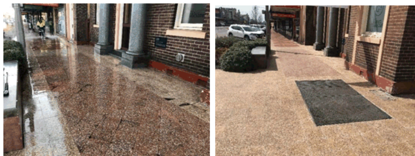
CBD Steam Cleaning – Before and After
