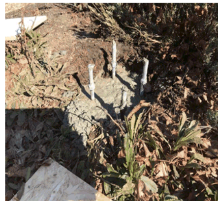
Footing for Flagpole
