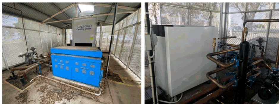
Civic Centre External Boiler – Old (Blue) and New
