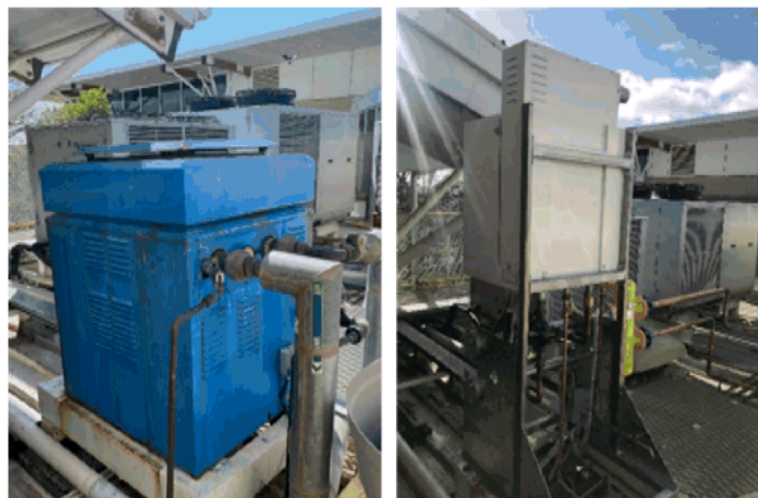
Civic Centre Internal Boiler – Old (Blue) & New
