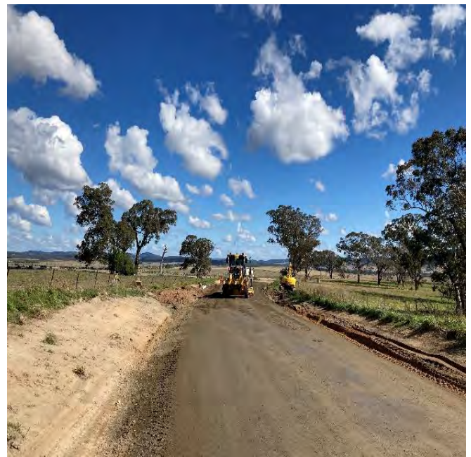
Sub base preparation of Stage 2
