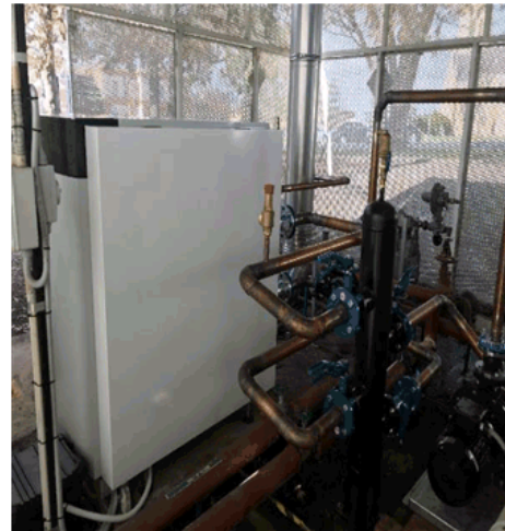
New external boiler
