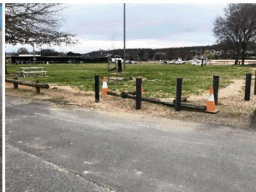
Log Replacement in Picnic Area
