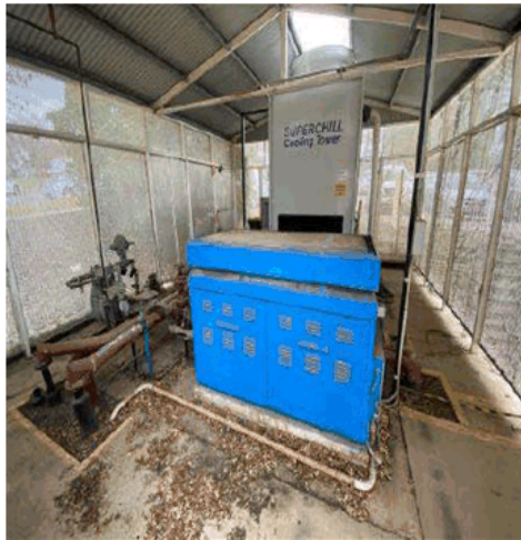
Old external boiler
