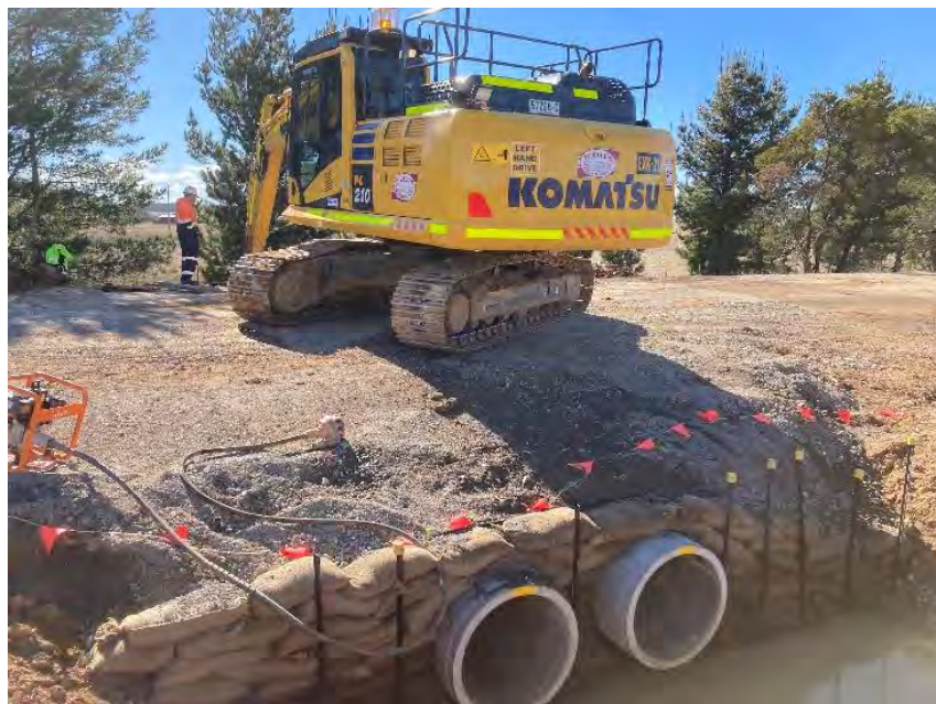
Duplication of existing drainage structure Stage 1
