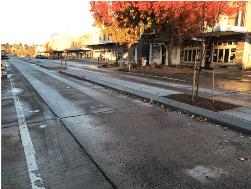
Auburn Median Replacement – Verner to Clinton Streets
