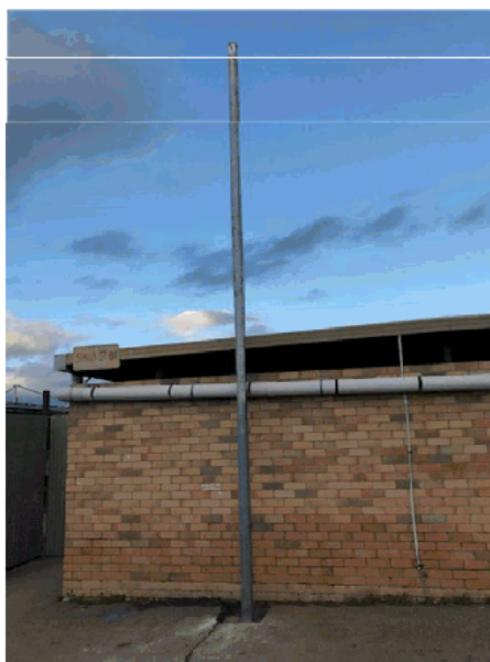
Goulburn Recreation Area -
