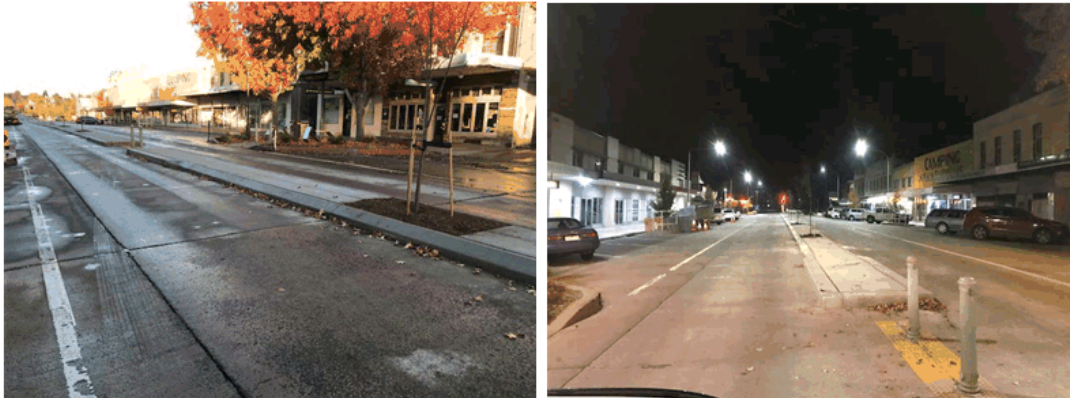
CBD Median Strip Replacement
