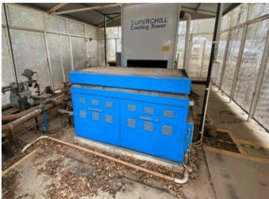
Main Boiler Civic Centre
