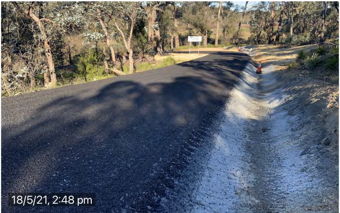
Works on Canyon Leigh Rd
