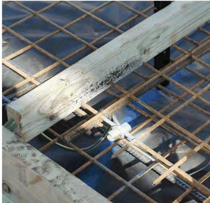
Electrical bonding connection to slab reinforcement mesh
