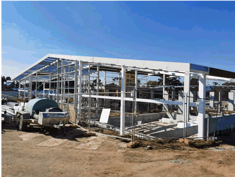
Structural Steel Framing
