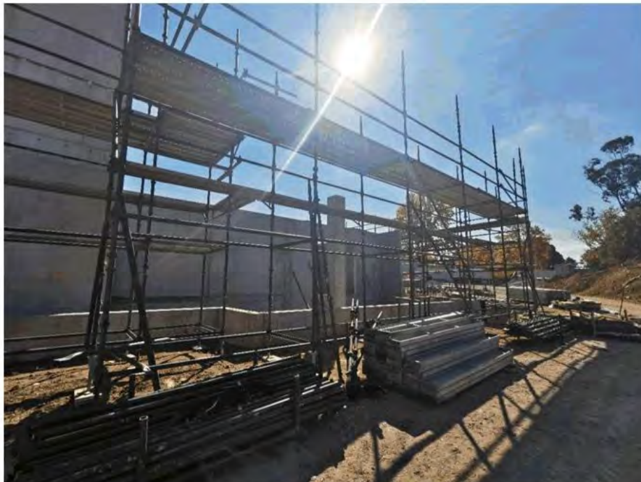
Scaffold installation in progress.
