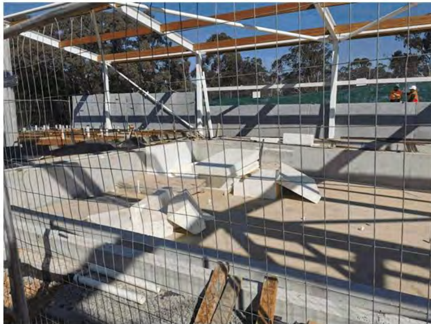
Indoor 25m heated lap pool progress
