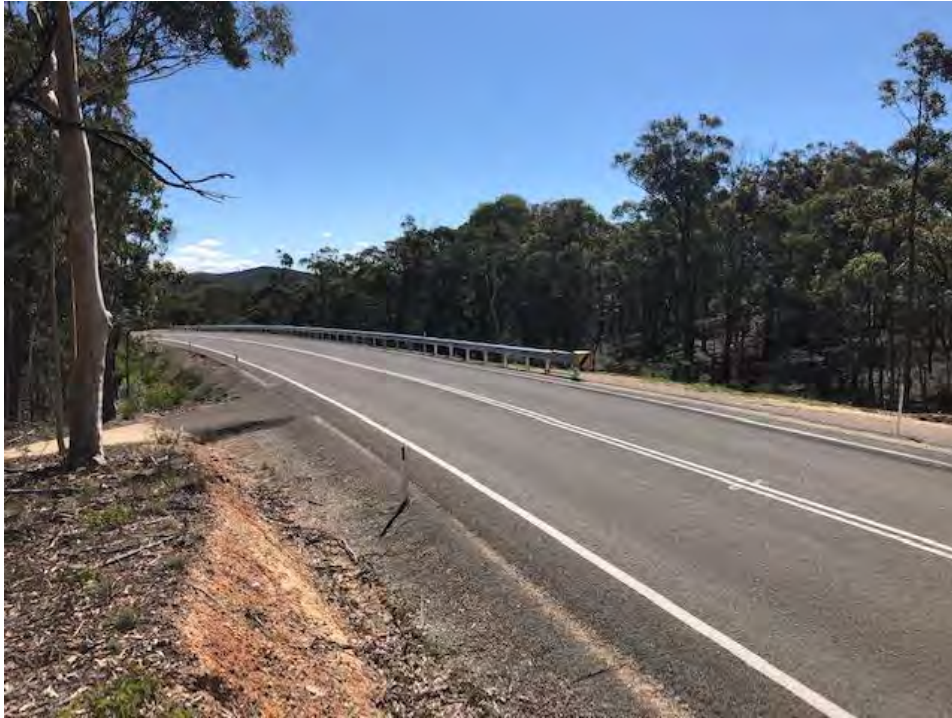
Guardrail installed on Mountain Ash Road
