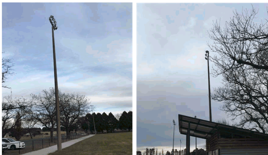
Eastgrove South Light Repairs
