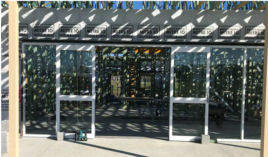
Cookbundoon Pavilion – Framing (prior to brickwork)
