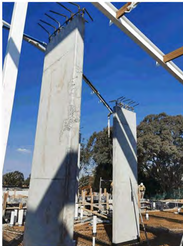
Structural Columns noting minor surface defects.
