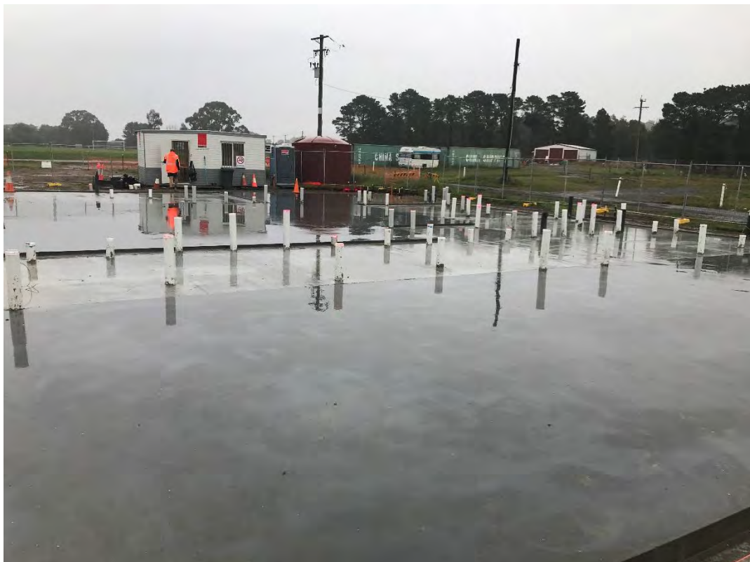
Installation of concrete slab
