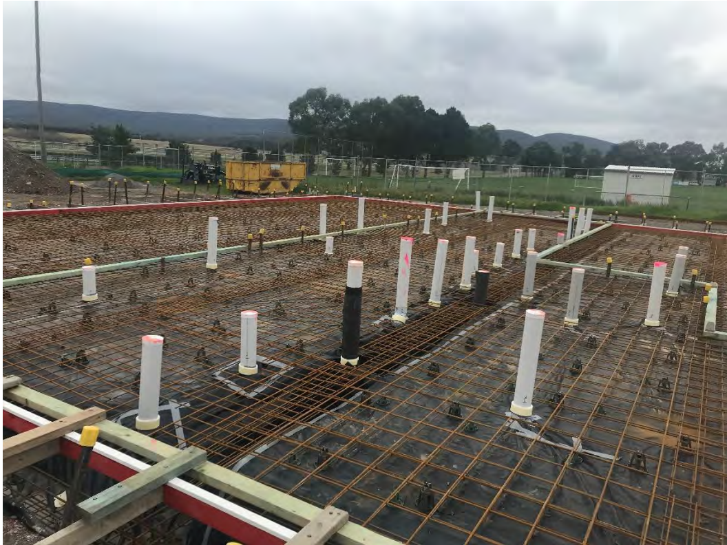
Cookbundoon Pavilion – Mesh and roughed in underground service protrusions.
