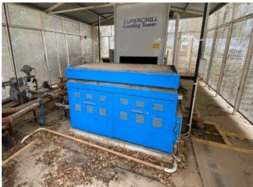
Main Boiler Civic Centre
