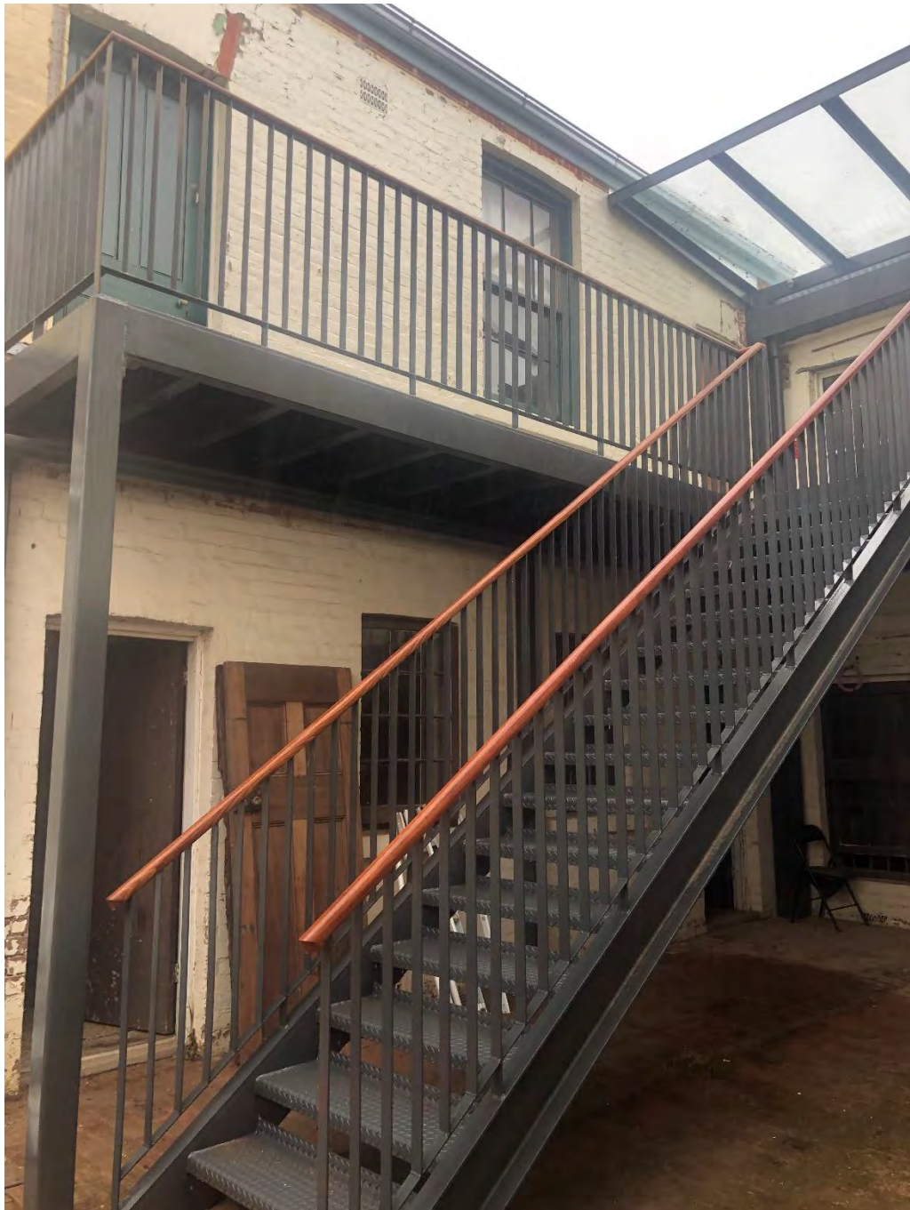
New Timber handrail installed on new stair and balcony at rear of St Clair Villa
