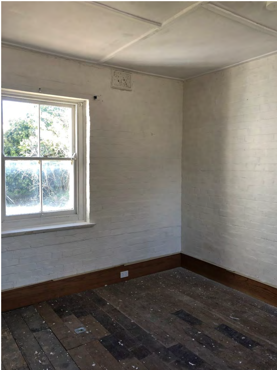
Interior painting of downstairs rooms in Coach house underway
