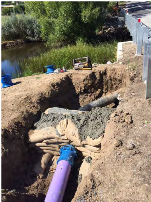
May Street Bridge Connection
