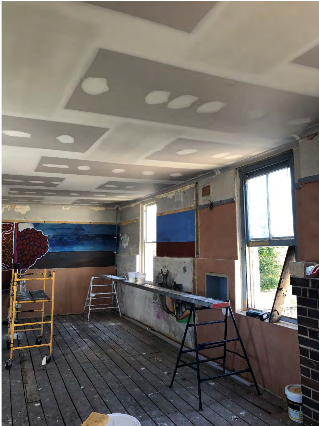
New ceiling being installed in Coach House
