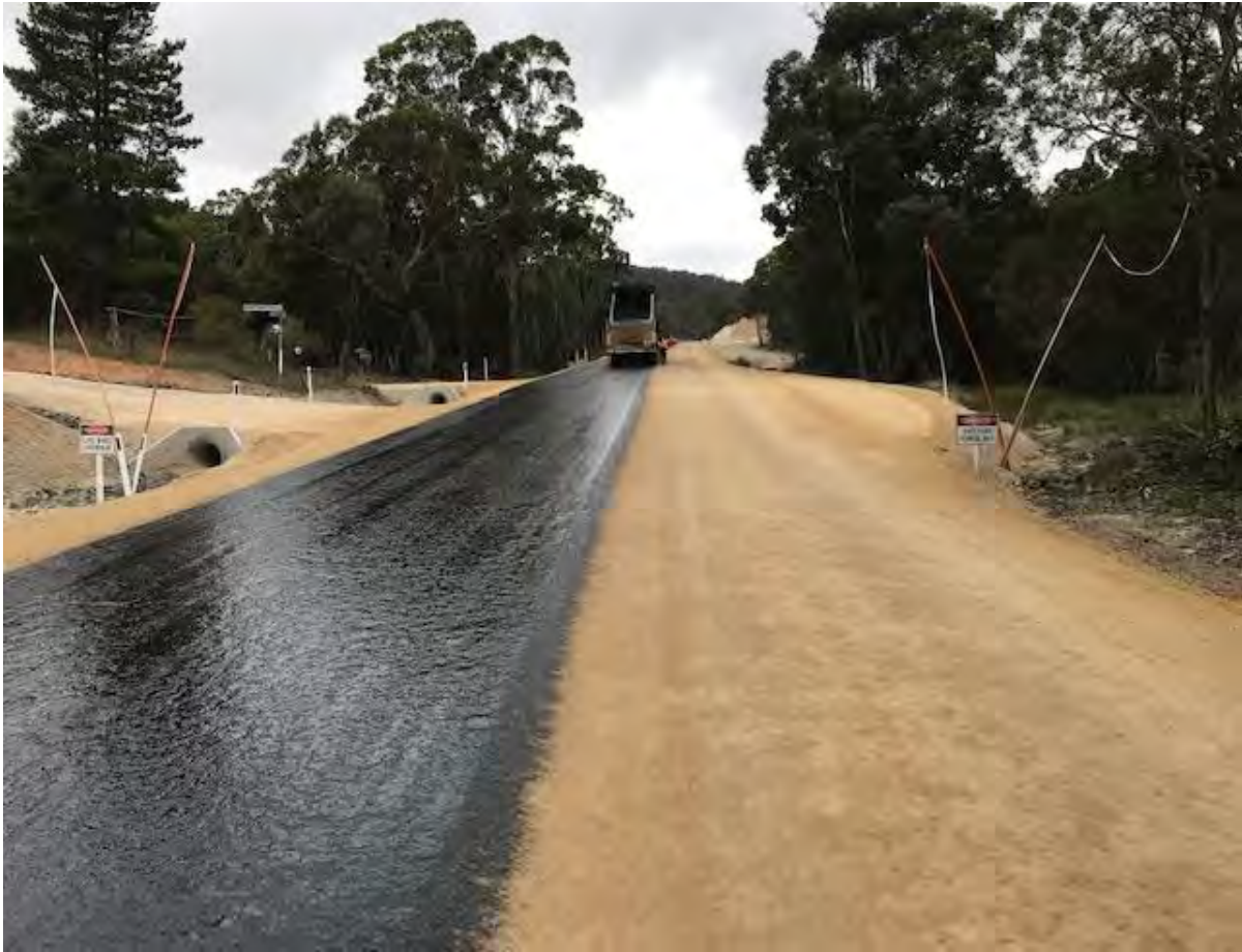
Bitumen sealing of the remaining 1.8km section of Mountain Ash Road
