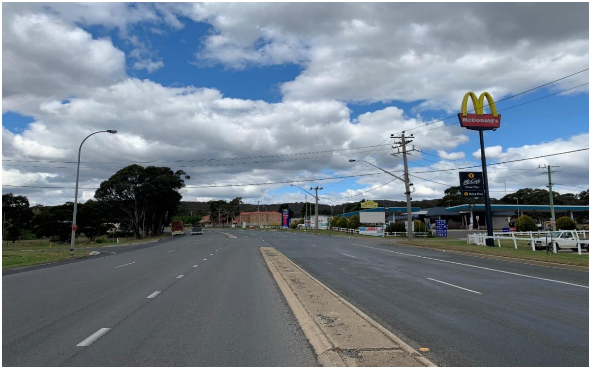
Sydney Road Eastbound
