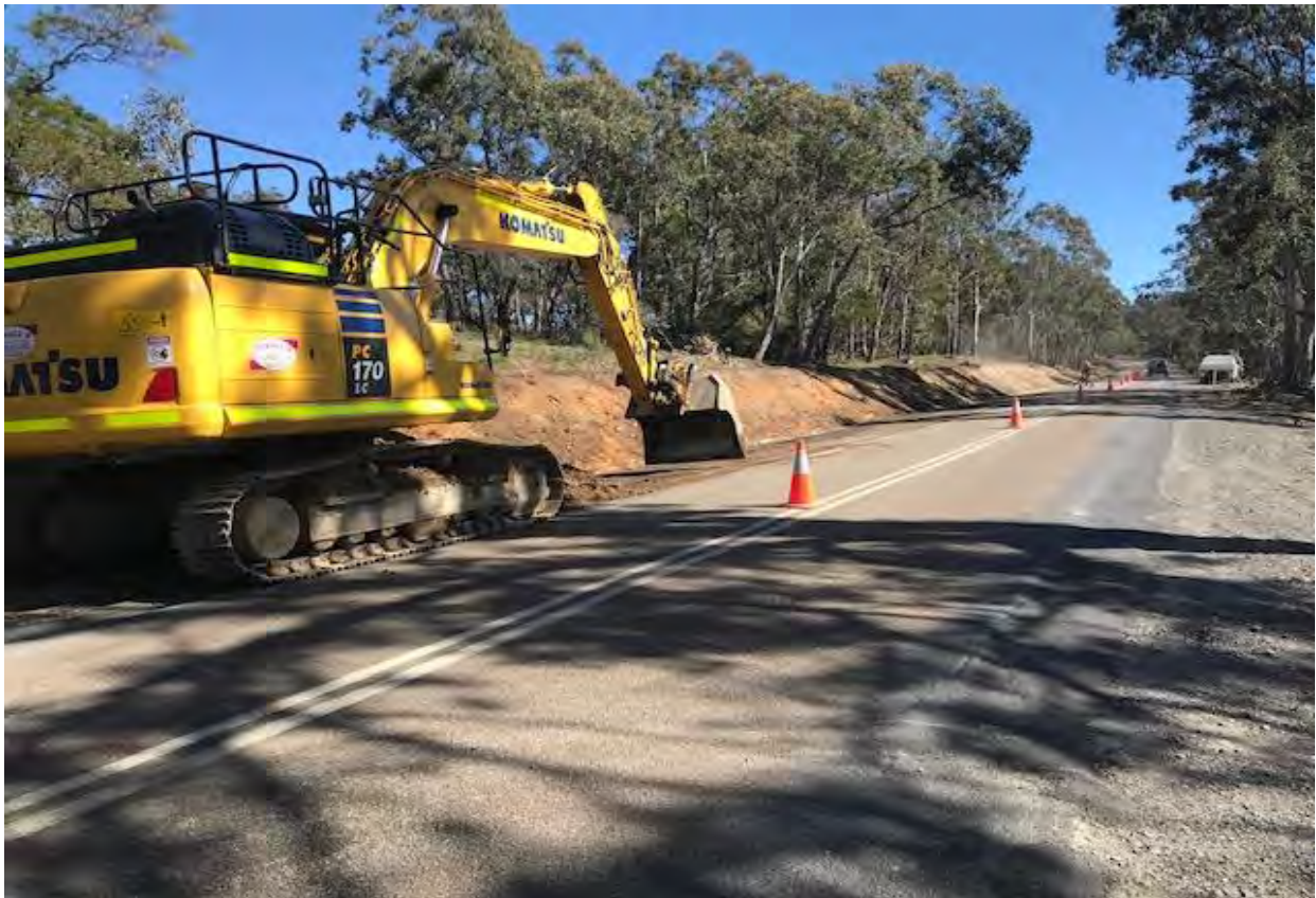
Batter and drainage works
