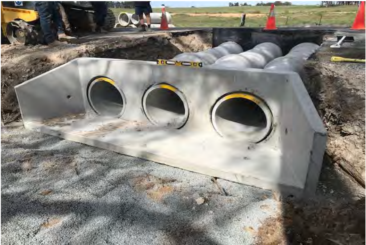
Triple Cell 600mm Culvert
