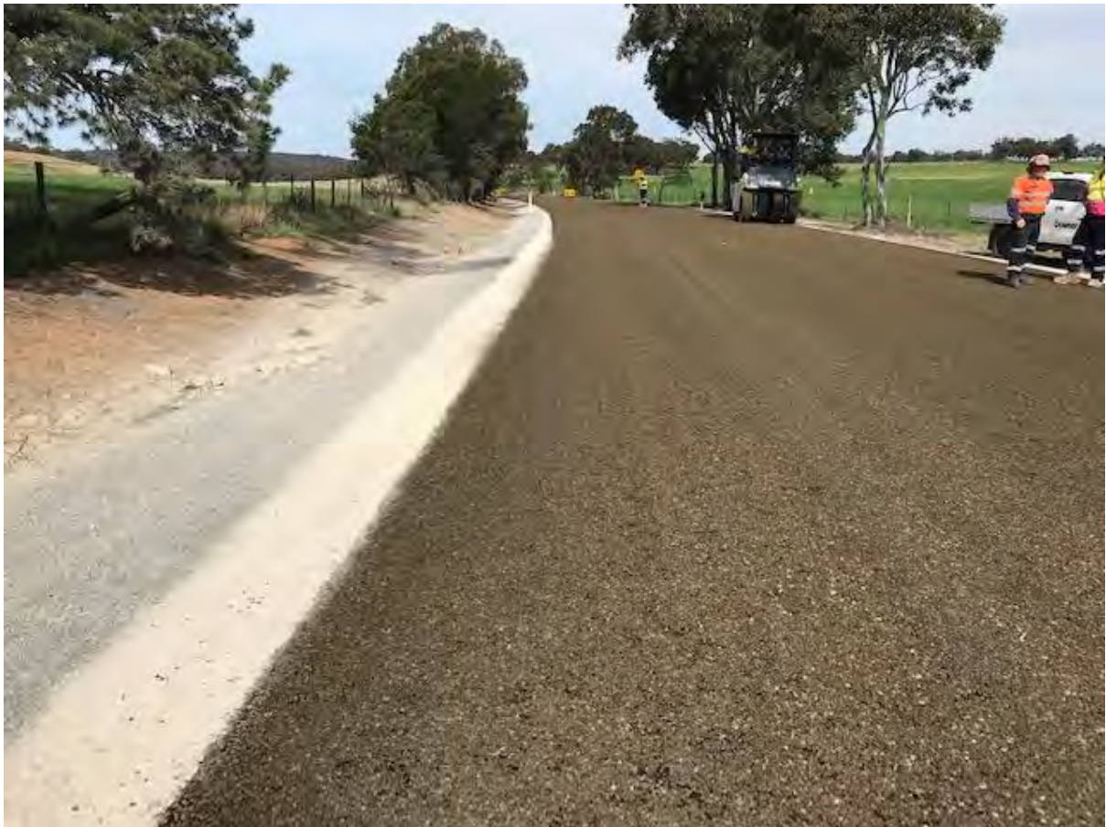
Stage 1 Mountain Ash two coat seal
