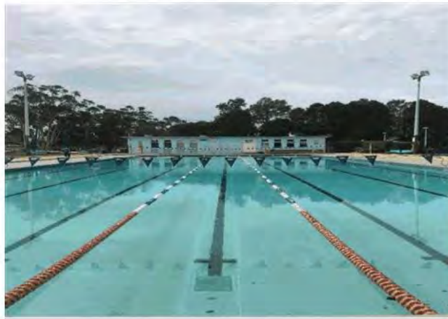
Outdoor Pool undergoing testing with the pool covers removed
