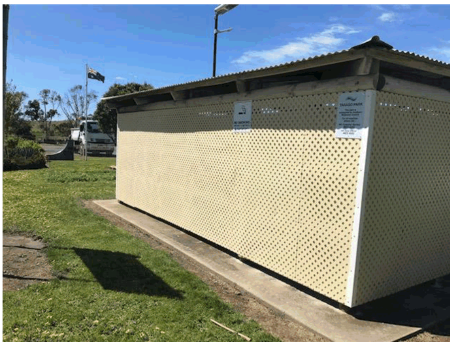
Tarago Picnic Shelter – after new cladding installed
