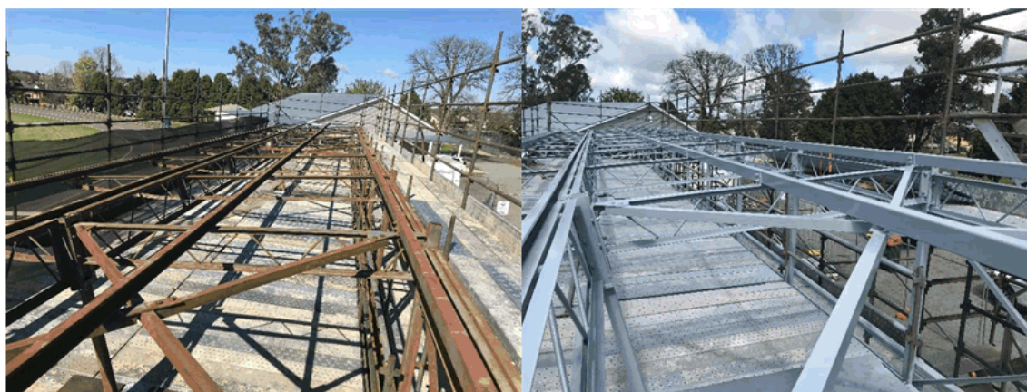
Max Hadlow Grandstand – before and after photos of roof beams painted
