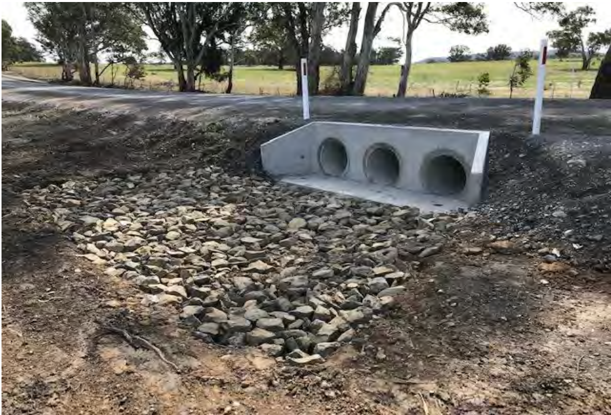
Completed culvert with gabion rock
