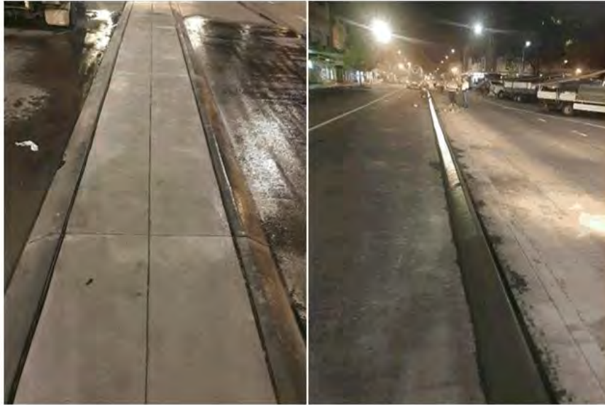
CBD Median Installation
