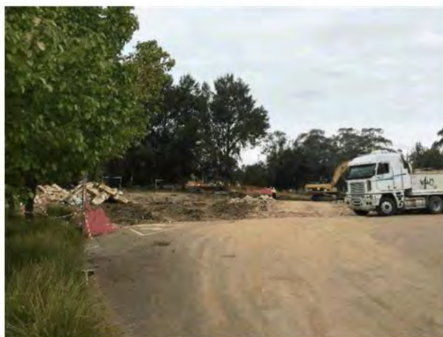
Demolition Site of Indoor Pool – Aquatic Centre
