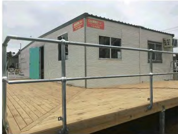
New site office entry – Aquatic Centre
