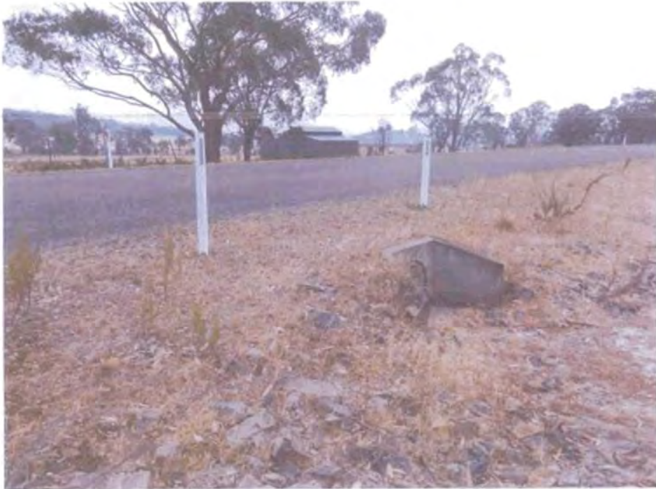
Storm Water pipe under Doisett Road looking north to 30 Doisett Road.
