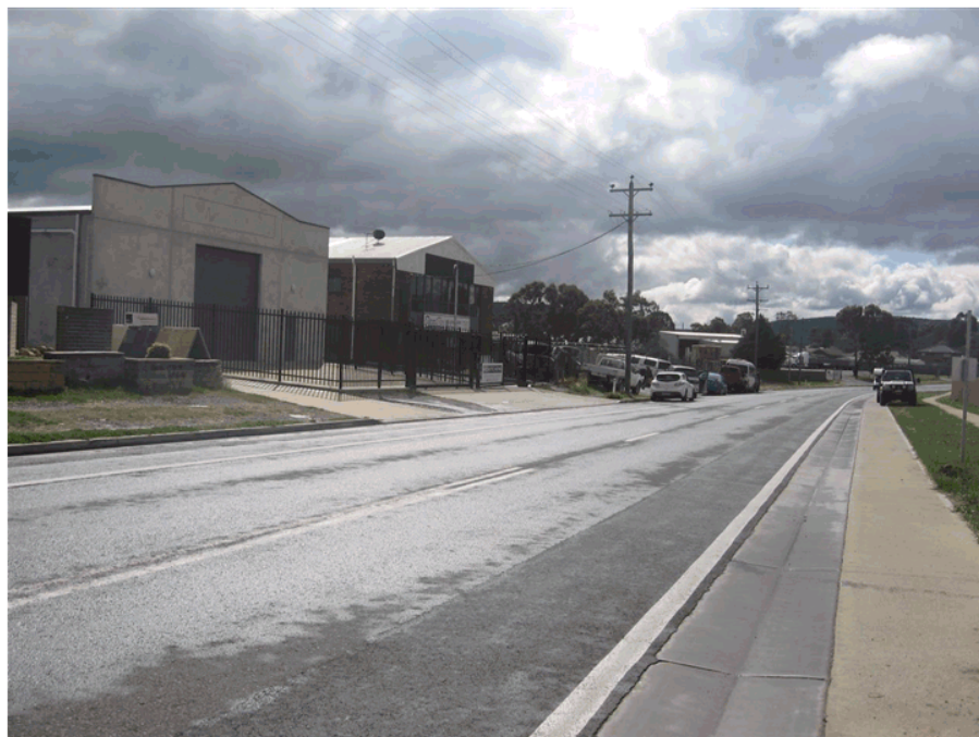
Existing Industrial Development – Taralga Road
