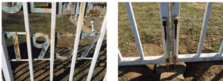
Photos of the cemetery gates show rust, paint deterioration and broken barrel bolts.
