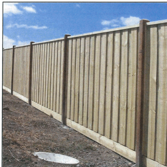
Typical Lapped and Capped Timber Fence
