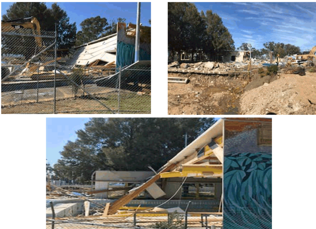
Photos of Indoor Aquatic Centre being demolished
