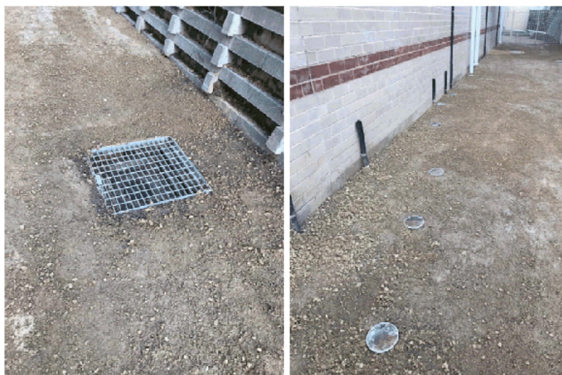
Sewer & Stormwater Pits Civic Centre
