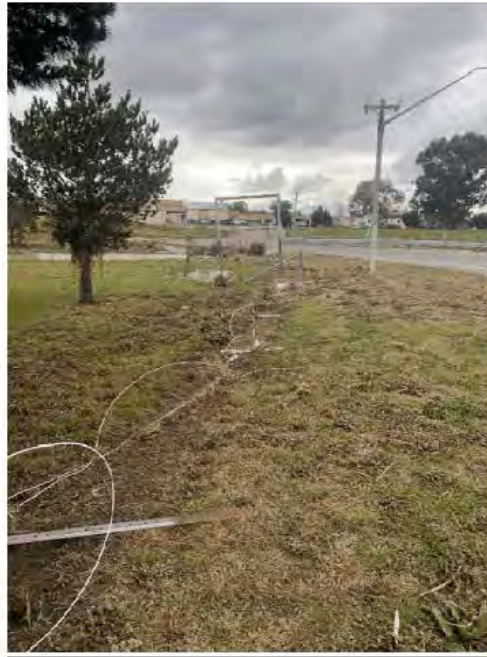
Damaged Fencing Park Road
