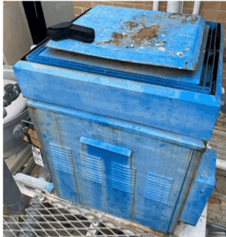
End of Life boiler
