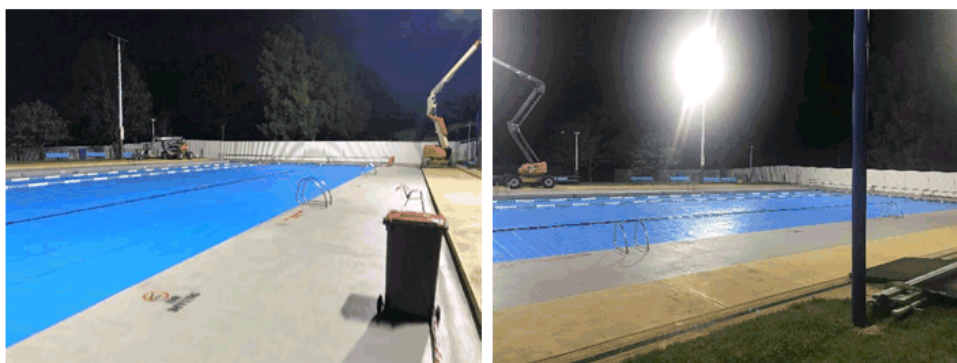
New Pool Lighting at the Goulburn Aquatic Centre
