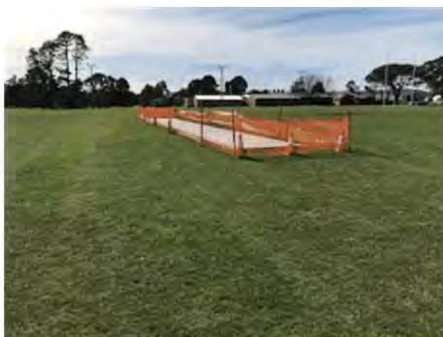
North Park – awaiting astro-turf and backfilling
