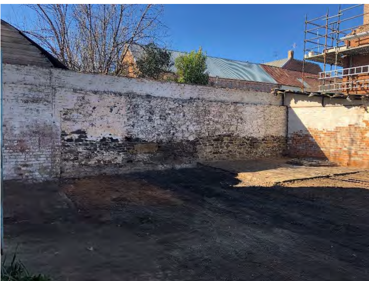
Demolition now complete. Sheds between the Villa and Coach House demolished.
