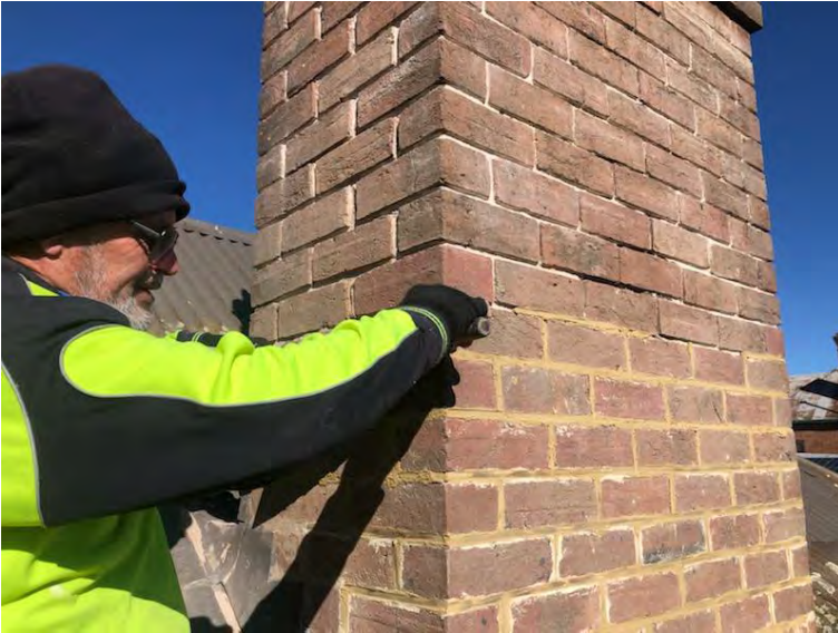
Re-pointing of chimneys on the Villa.
