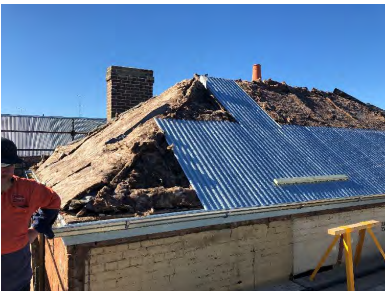
New roof being installed at rear, using short sheets as was the original heritage method.
