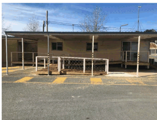
Hetherington Street Depot – Meal Room / Training Room Ramp
