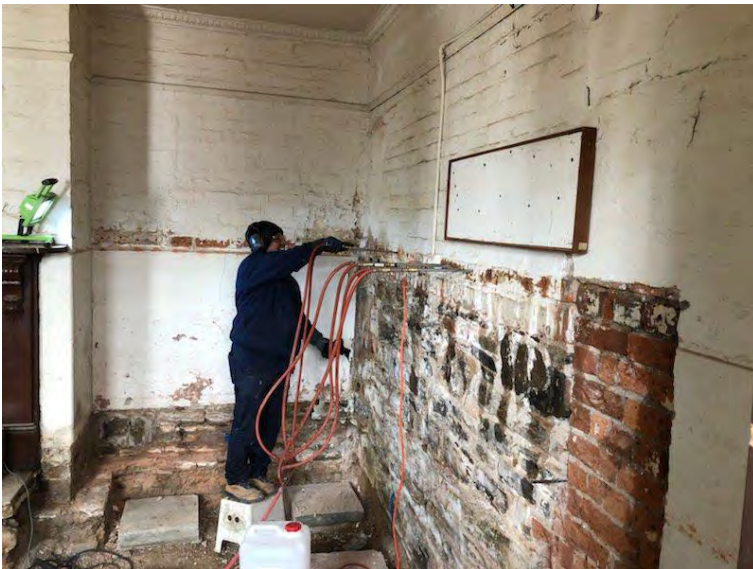
Damp proof injection underway in ground floor rooms.
