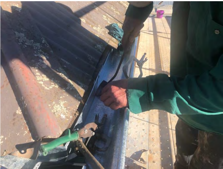
New gutters being installed using traditional methods
