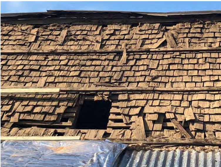
Image of original shingled roof prior to new roof being installed.
