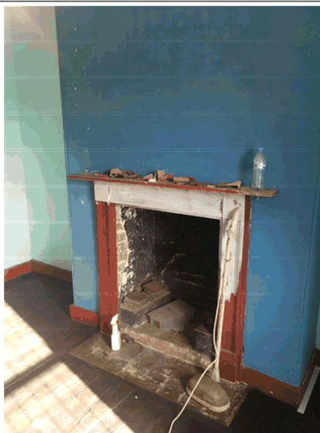
Photo 30 – Condition of existing fireplace in Bedroom 3.
