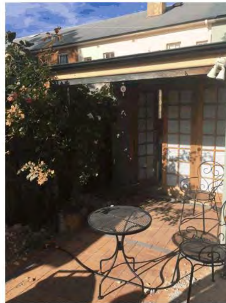
Photo 6 – Verandah along with structure, roofing, gutters & fascia, triple-leaf door and brick paving.
