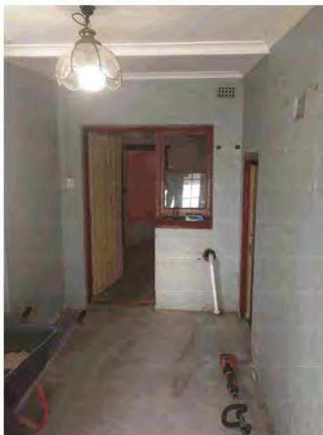
Photo 7 – Existing brick walls, with door and window at rear of building.
