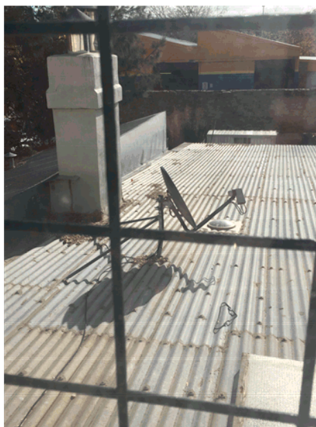
Photo 32 – Overall condition of existing ground level roof and services.
