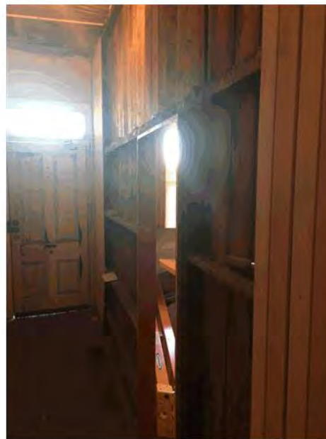
Photo 20 – Condition of existing timber clad wall in entry.
