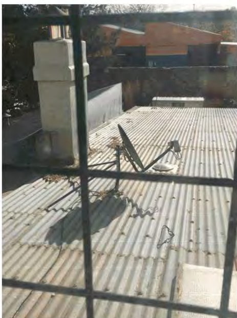
Photo 15 – View of existing roof services, chimney to kitchen fireplace and roof to ground floor.
