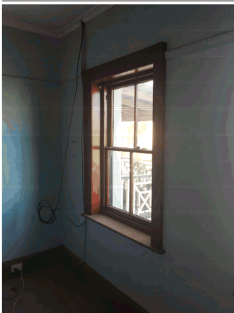
Photo 29 – Condition of walls and window in Bedroom 2.
