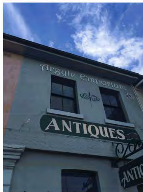
Photo 4 – External view of, eave and gutter, and windows to upper floor of building.
