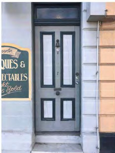
Photo 3 – External view of entry door at front of building.
