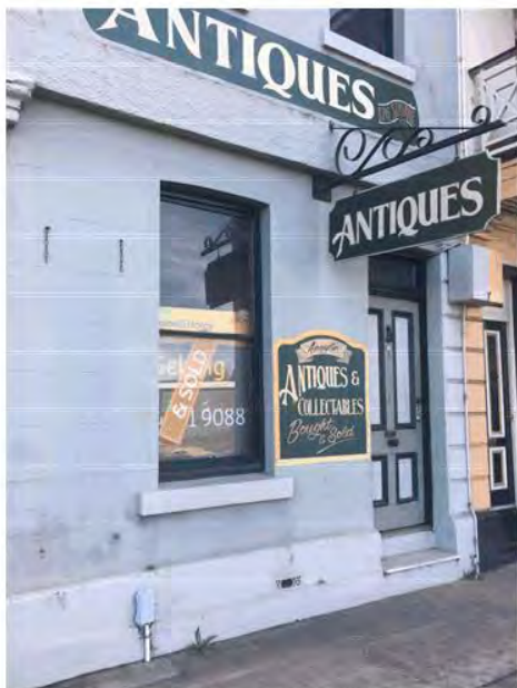
Photo 1 – External view of window and signage at front of building.
