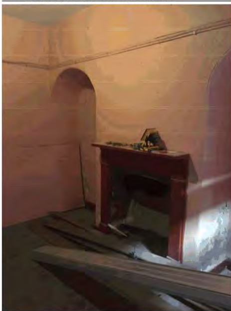
Photo 21 – Overall condition of walls, skirting and flooring in living room.
