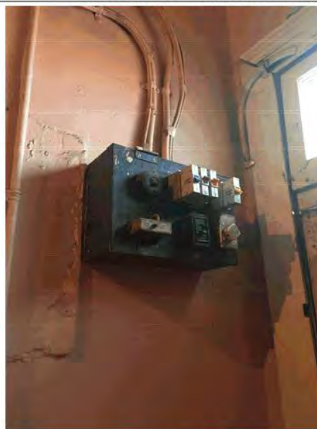
Photo 14 –View of existing electrical living area. switch box at front entry door.
