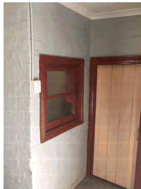
Photo 8 – View of window to bathroom/laundry and door to existing wash closet.
