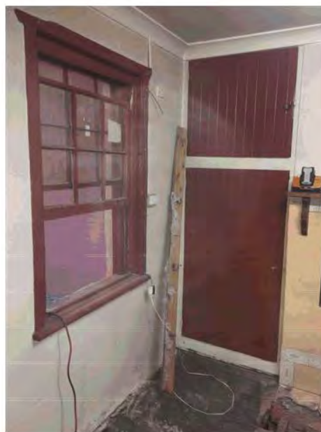
Photo 24 – Existing internal window between bathroom and kitchen.
