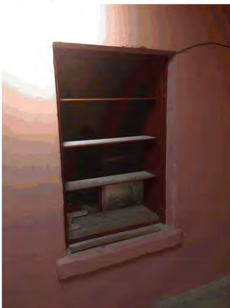
Photo 23 – 1 of 2 existing openings in bathroom.
