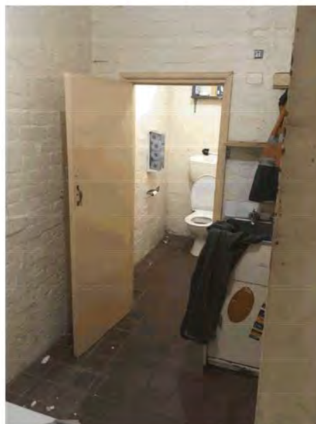
Photo 10 – View of laundry tub and view into wash closet from bathroom/laundry at rear of building.
