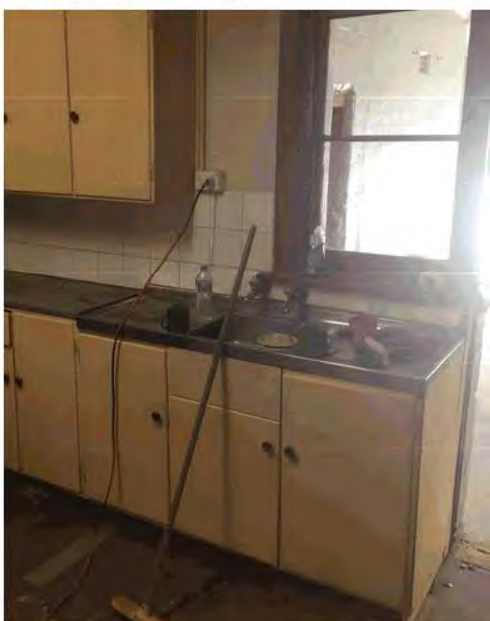
Photo 11 – View of casework, sink, window and floor condition in kitchen at rear of building.
