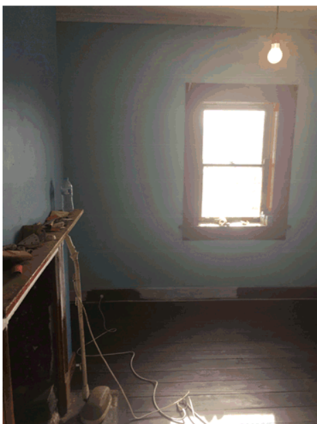
Photo 31 – Overall condition of walls, skirting, fireplace and window in existing Bedroom 3.
