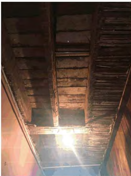
Photo 19 – Condition of ceiling in entry.
