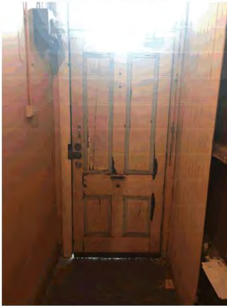
Photo 17 – Internal side of entry door.
