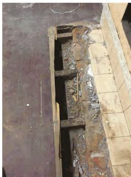
Photo 12 – View of timber floor structure in kitchen.
