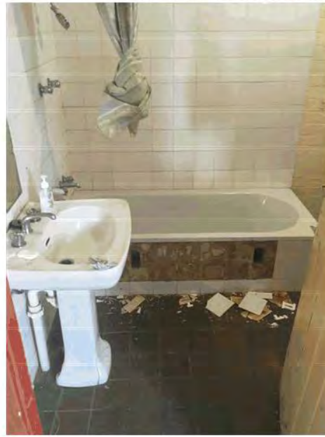
Photo 26 – Condition of existing bathroom.
