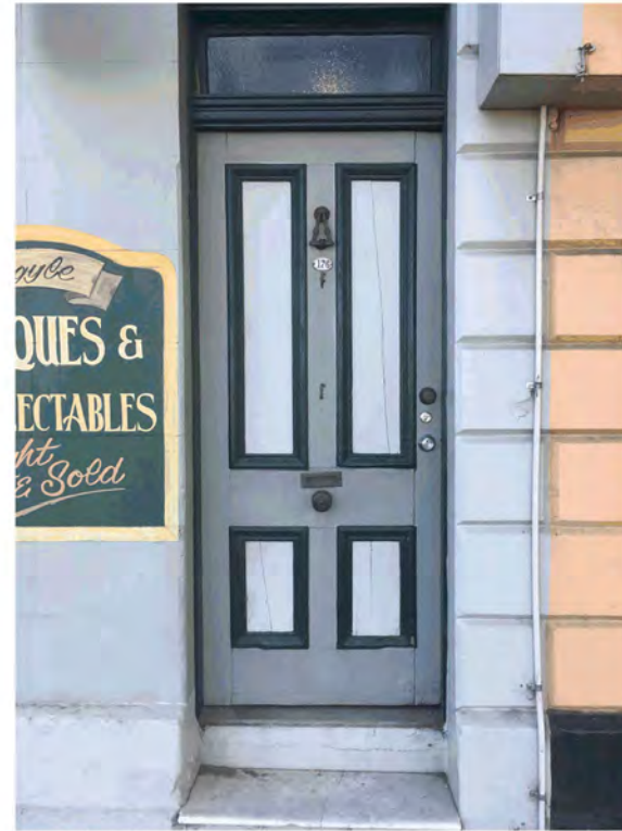
NEW EXTERNAL DOORS TO BE PAINTED TO MATCH EXISTING TERRACE. DESIGN TO MATCH EXISTING AS CLOSELY AS PRACTICALLY POSSIBLE.
