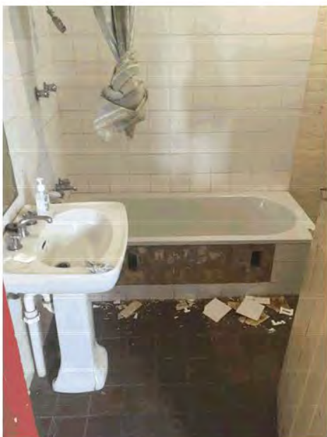
Photo 9 – View of washbasin & bathtub in bathroom/laundry at rear of building.
