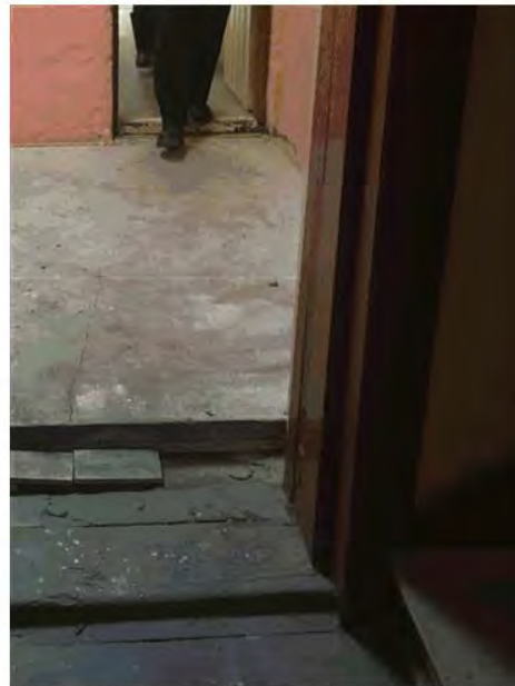
Photo 28 – Level change between living room and bathroom slab.
