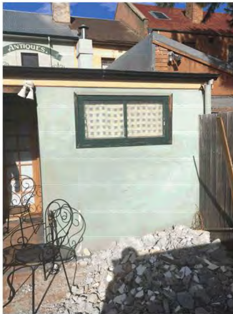
Photo 5 – Existing storage & timber boundary fence.
