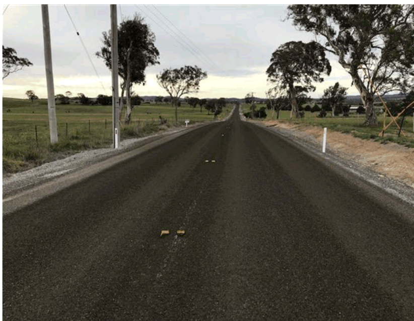
Middle Arm Road widening & bitumen over seal
