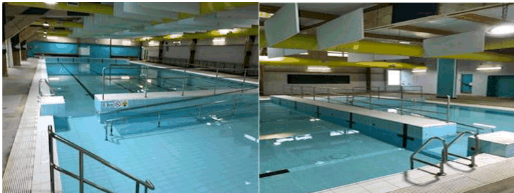
Indoor Pool Ready for Demolition
