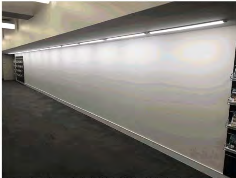
Library shelving removed and wall painted
