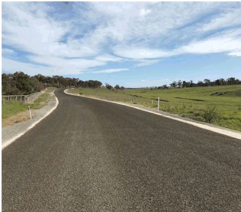
Range Road – bitumen over seal
