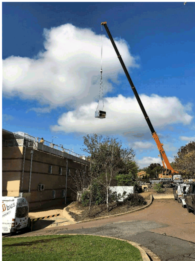
Civic Centre Air Handling Unit Installation
