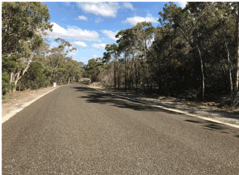
Taralga Road – Bitumen over seal
