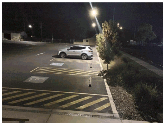
New Lighting – Hetherington Street Car Park
