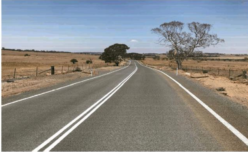
Gurrundah Road rehabilitation
