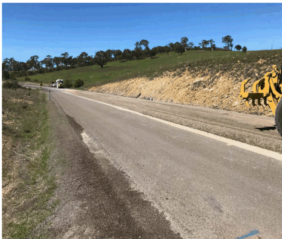
Range Road pavement stabilisation
