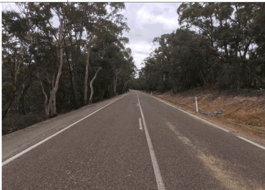
Taralga Road drainage & edge works
