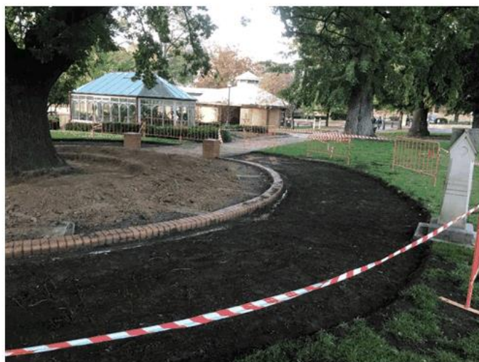
Belmore Park – Work commencing on the Lady Belmore Tree.
