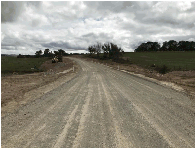
Curve re alignment on Pomeroy Road
