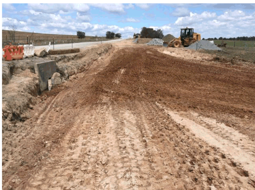
Curve realignment - Pomeroy Road
