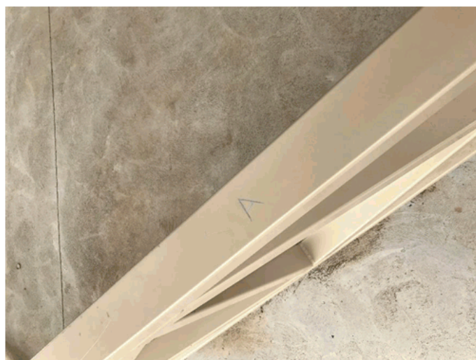
Rotary Park – Vandalism
