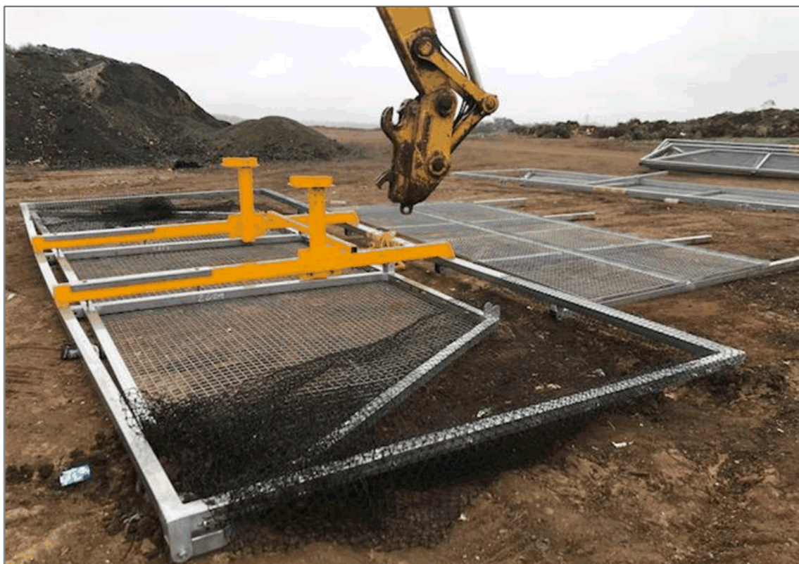
Photo: New litter nets being constructed at Goulburn Waste Management Centre.
