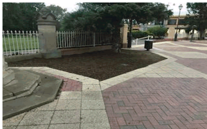
Belmore Park – Mulch Installed
