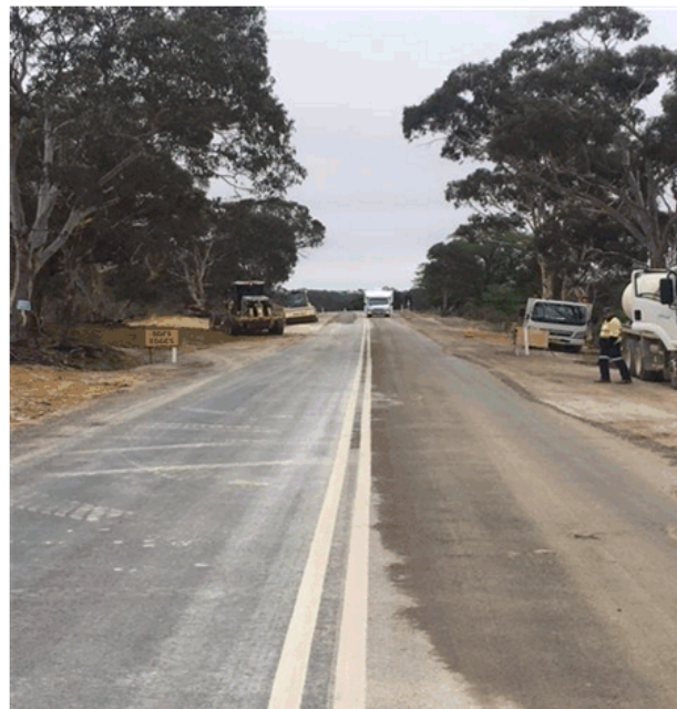
Range Road widening
