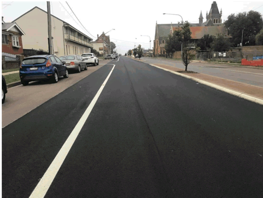
New asphalt on Bourke street
