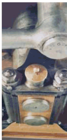
Before – oil well lid in place
