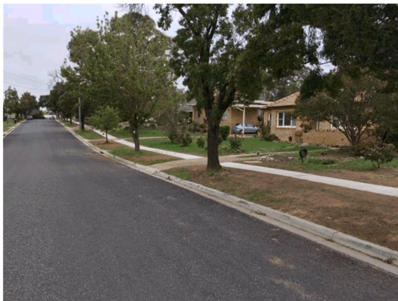
Rhoda Street – need photos of new footpath
