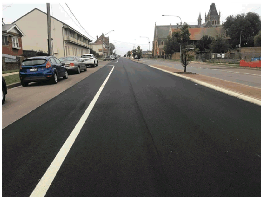
New asphalt on Bourke street
