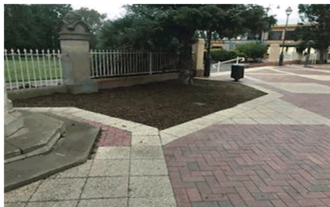
Belmore Park – Mulch Installed
