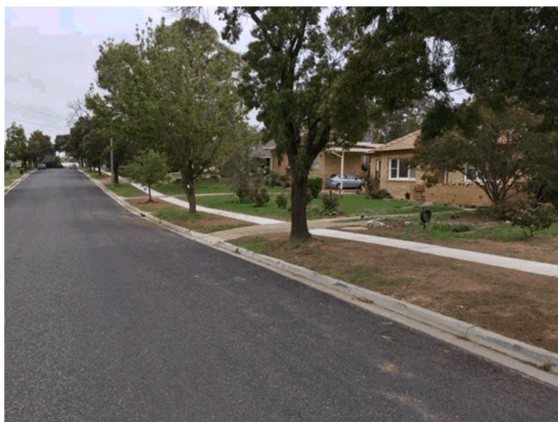
Rhoda Street – need photos of new footpath
