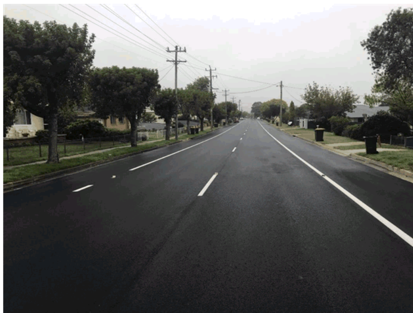
Taralga Road asphalt
