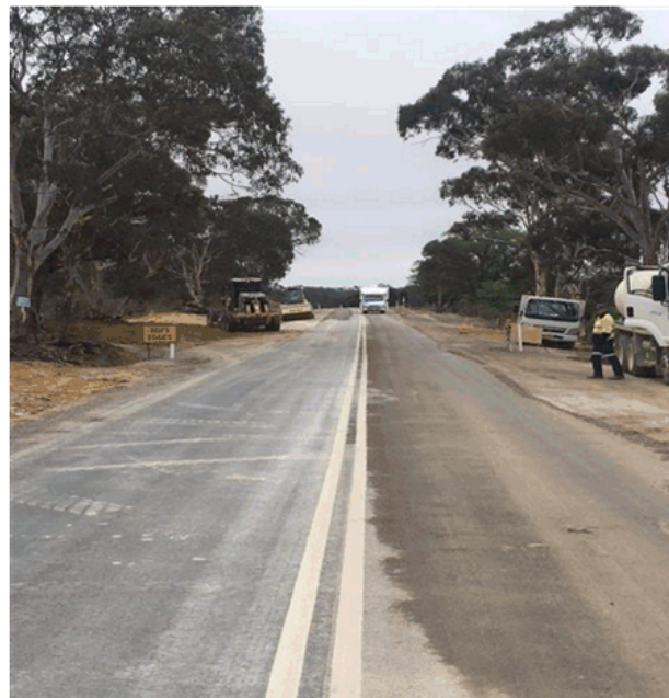
Range Road widening
