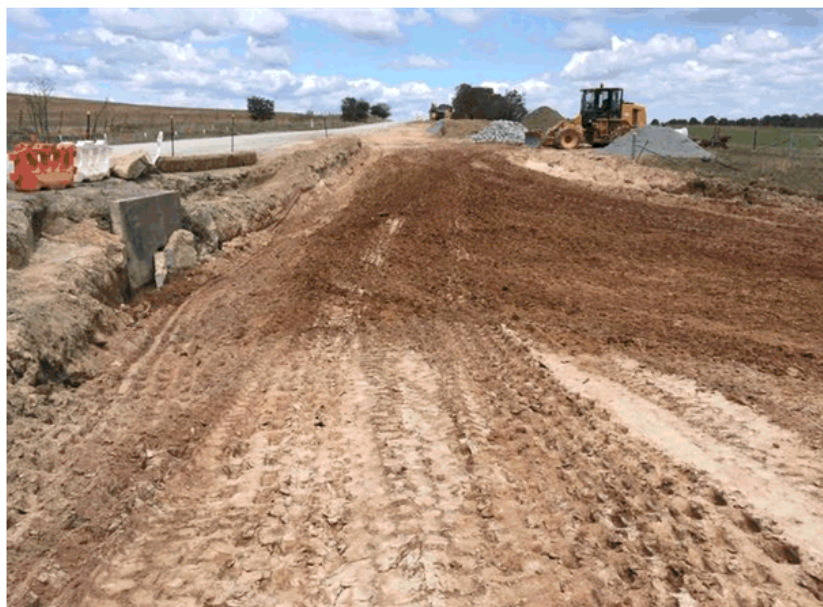
Curve realignment - Pomeroy Road
