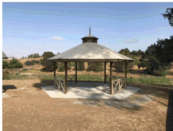
Rotary Park – newly installed rotunda
