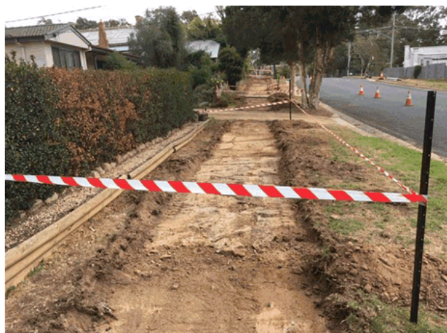
Rhoda Street - footpath excavation
