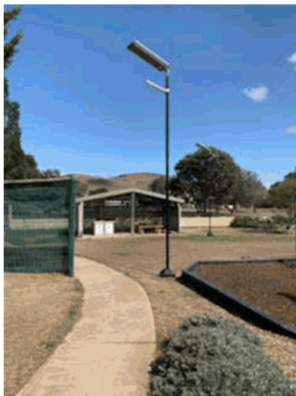
Tarago Park – newly installed solar lights
