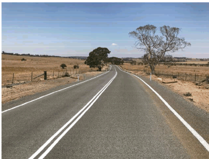
Gurrundah Road – Pavement rehabilitation
