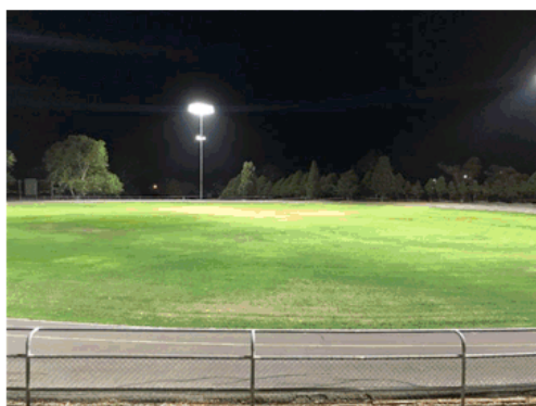
Seiffert Oval Lights - view from Clubhouse to the centre of the field
