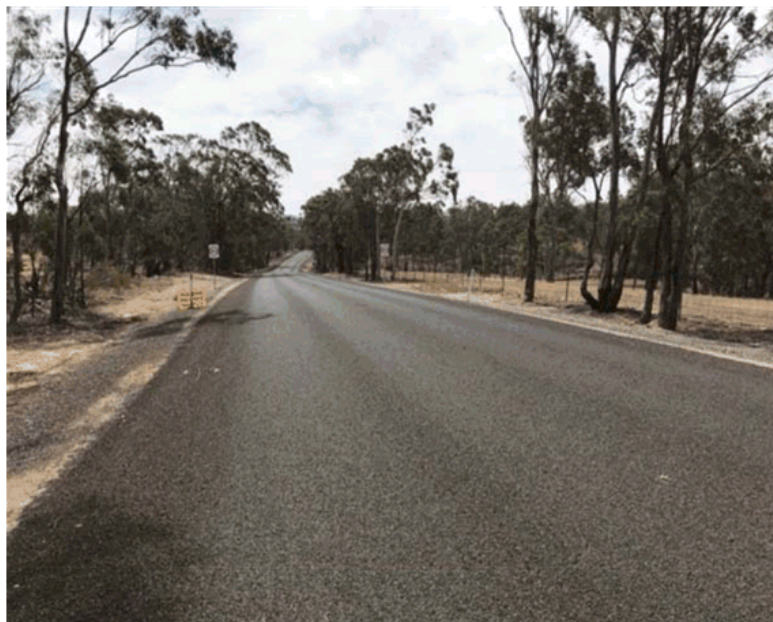
Oallen Ford Road Resealing Prior to Line Marking
