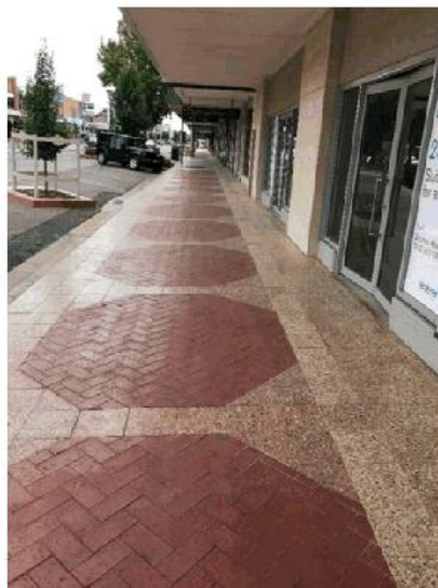
CBD Pavement after resealing – eastern side Montague Street to Clinton Street
