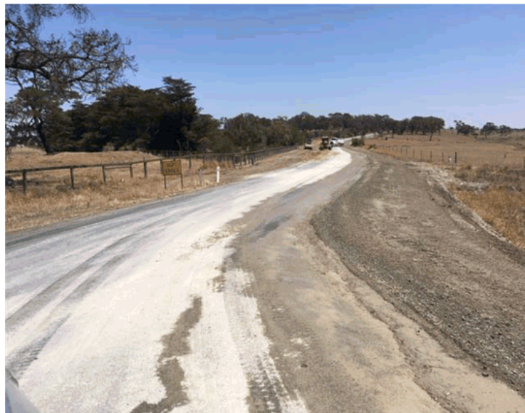
Range Road, shoulder widening at Baw Baw Road
