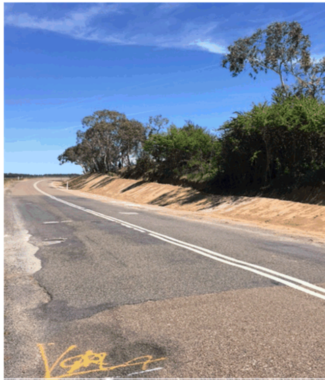
Gurrundah Road – preliminary drainage works
