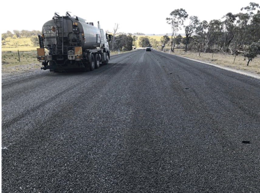
Haulage Route Re Sealing - Bitumen spray sealing Brayton Road
