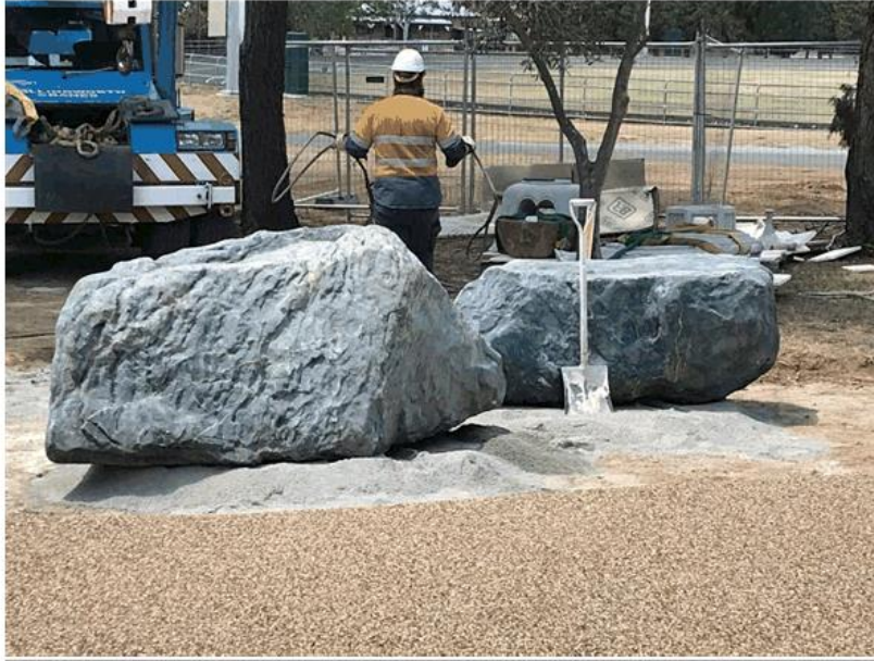
Staff and contractors placing the Shibetsu Boulders in place
