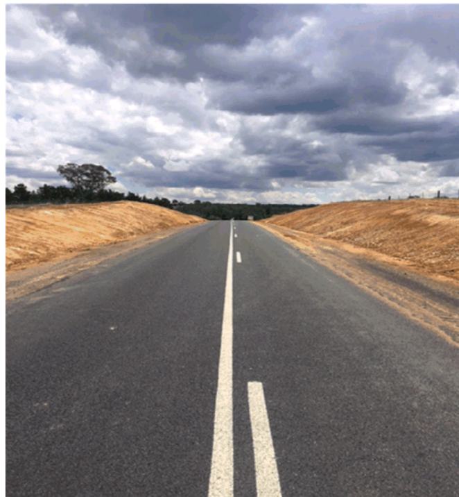
Range Road – Preliminary drainage works
