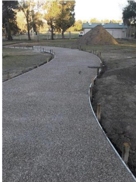
Path leading to entrance.
