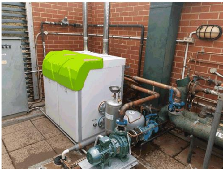
Meridian Condensing Units similar to those being installed in 50m pool
