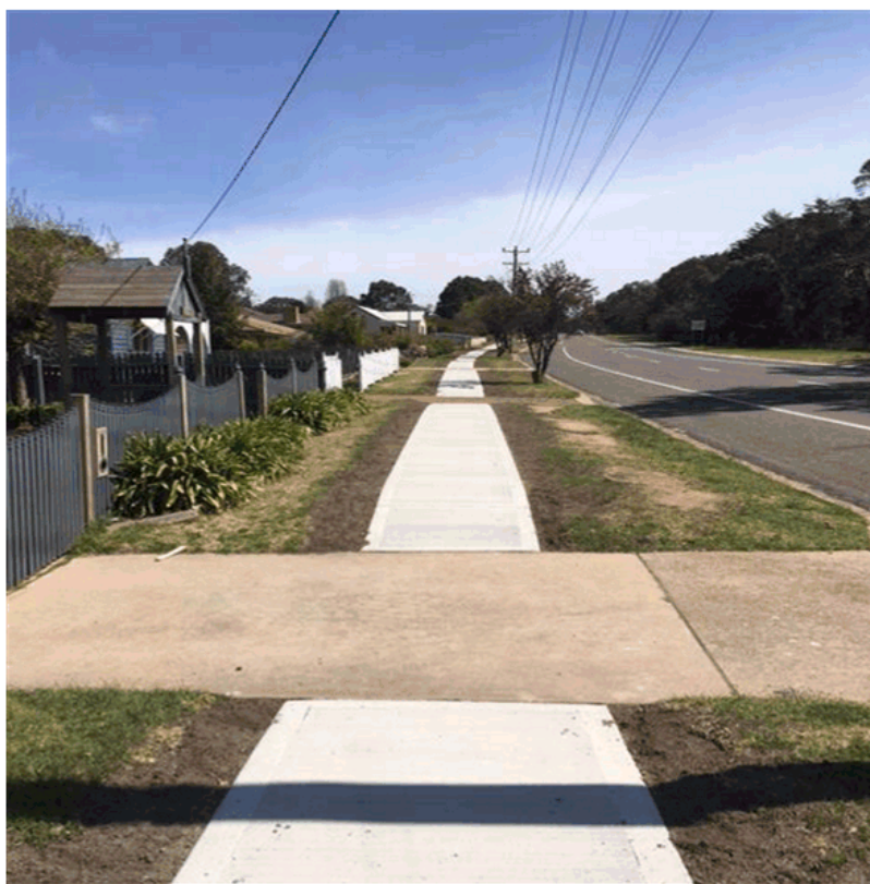
New footpath along Addison Street between Coinda Street and Duke Street
