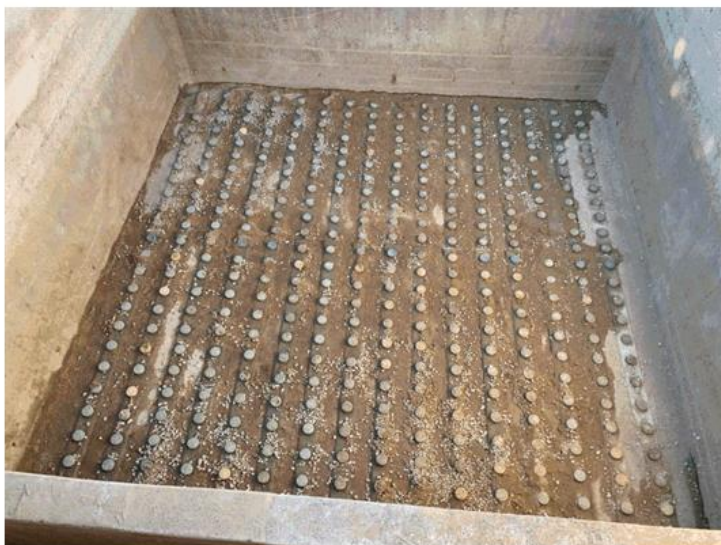
Cleaned out Sand Filters – 50m Outdoor Pool
