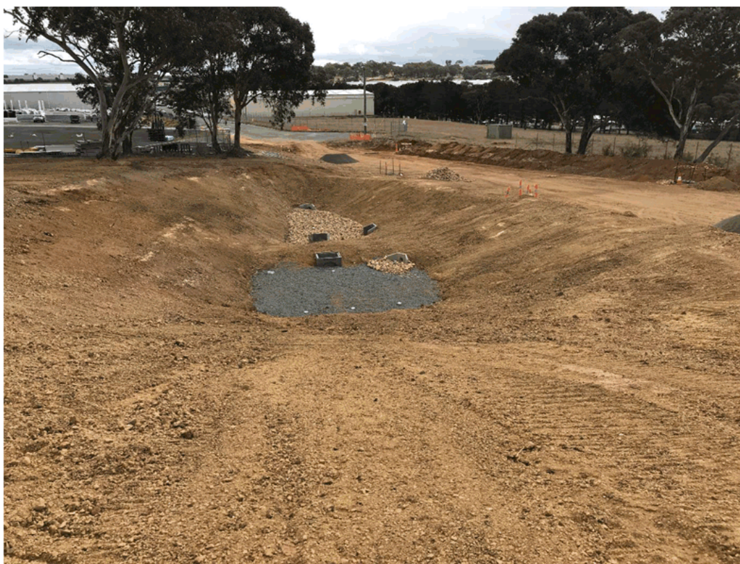
Lockyer – Storm water detention basin
