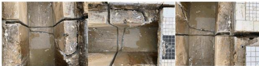
After removing old joint and putty used on old repairs.
