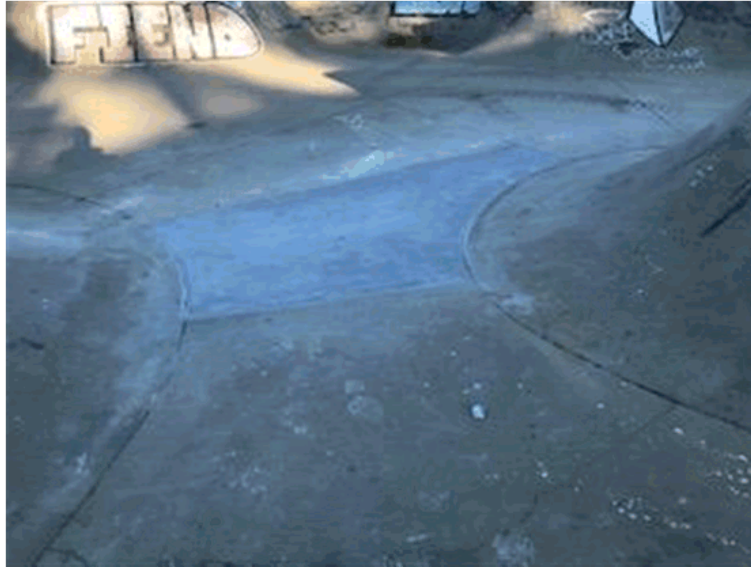
Victoria Park Skate Park Slab Repair
