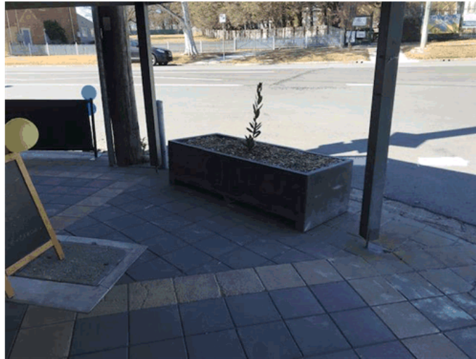
One of the new pots installed on the corner of George and Goulburn Streets
