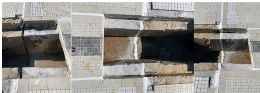
After new repairs and replacement joints
