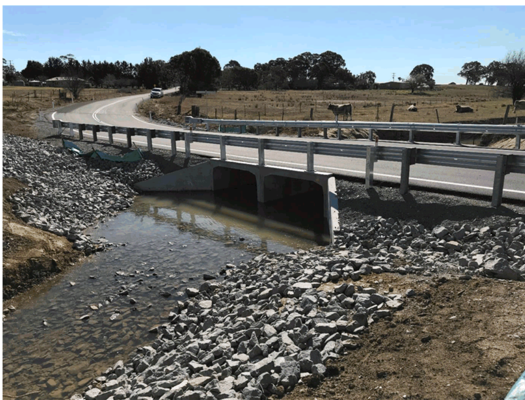
Parkesbourne Road – completed project
