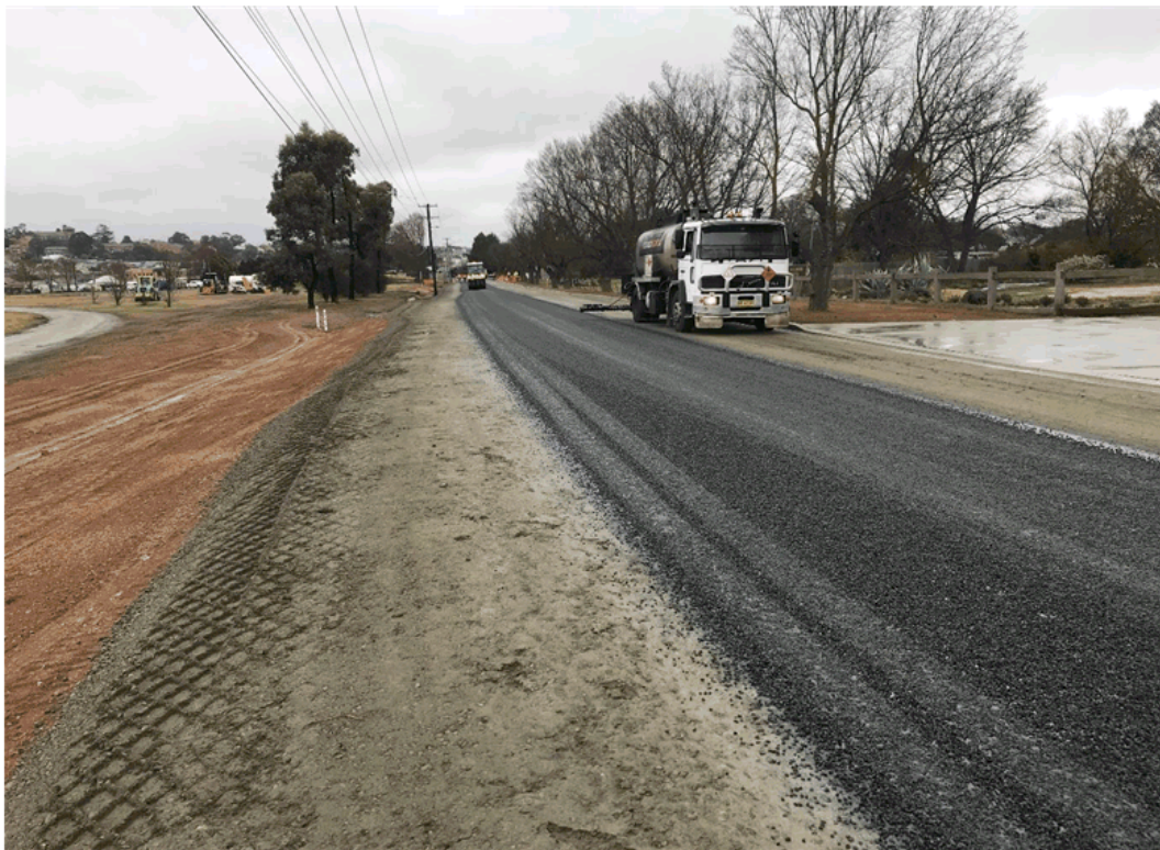
Bungonia Road – Prime sealing
