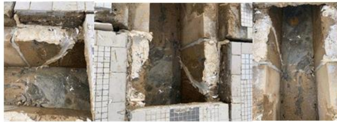
Joint condition on first look.
