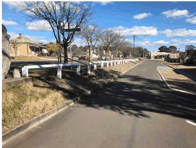
Freshly painted guard rail – frontage of Tony Onions Park
