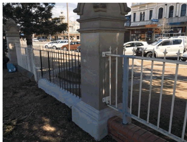
Belmore Park – Auburn Street Fence Restoration
