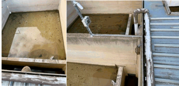
Existing Sand Filters
