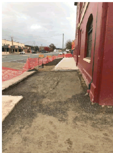
Sloane/Clinton Streets construction work underway
