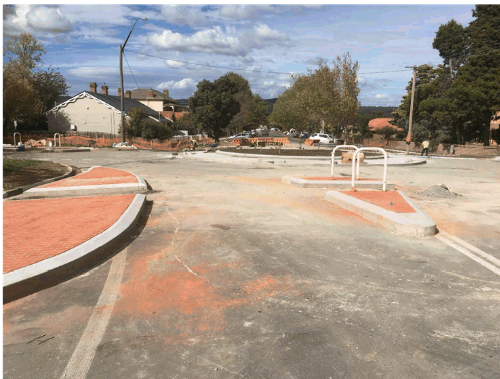
Roundabout nearing completion
