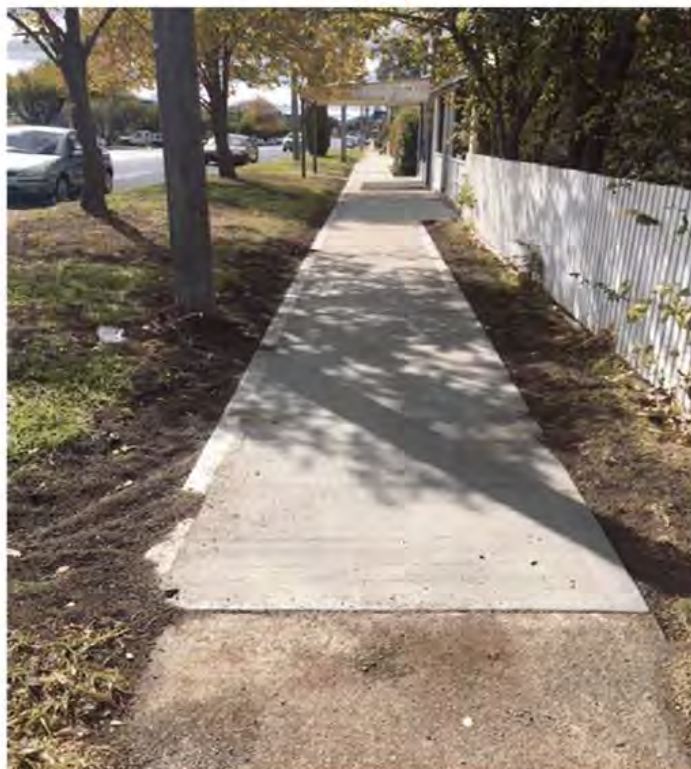
New footpath from Glebe Street to Walker Street
