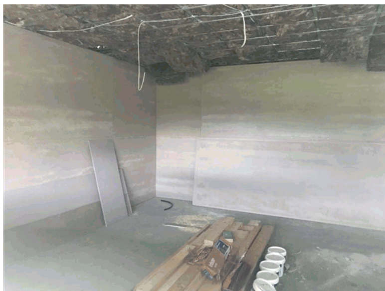
Internal walls and installation within Sporting Pavilion
