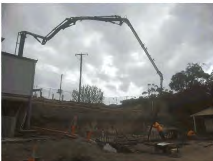
Pouring concrete footings
