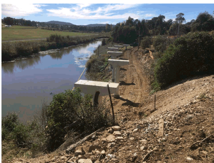
Elevated footpath under construction
