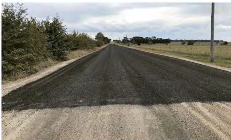
Highland Way heavy patching and overlay with seal
