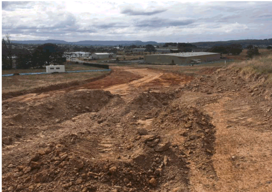
Tait Lockyer earthworks - Stripping of topsoil
