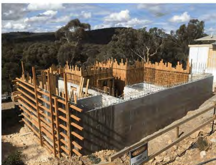
Concrete wall under construction
