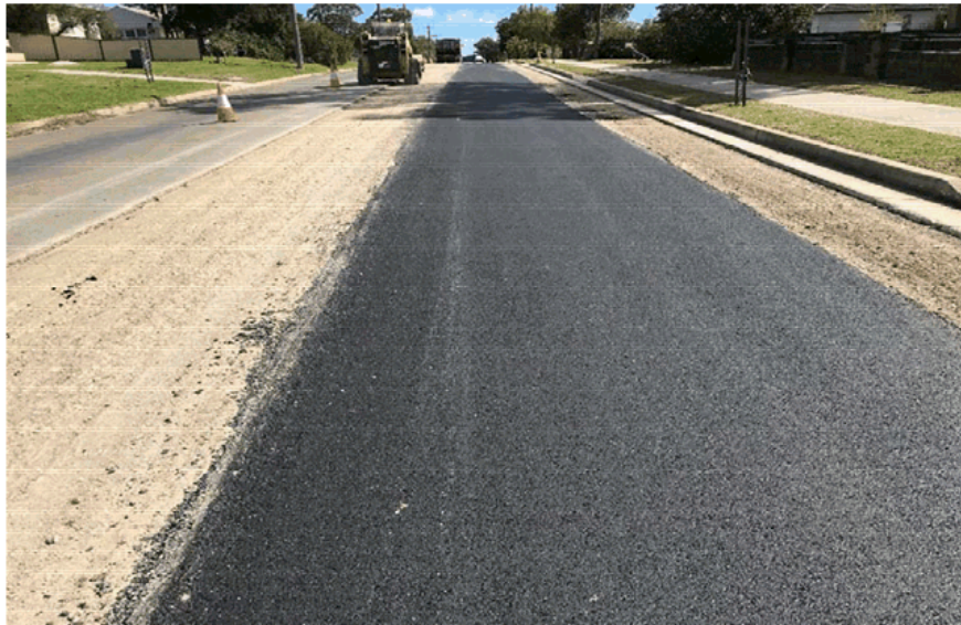
Brayton Road milling and placing AC
