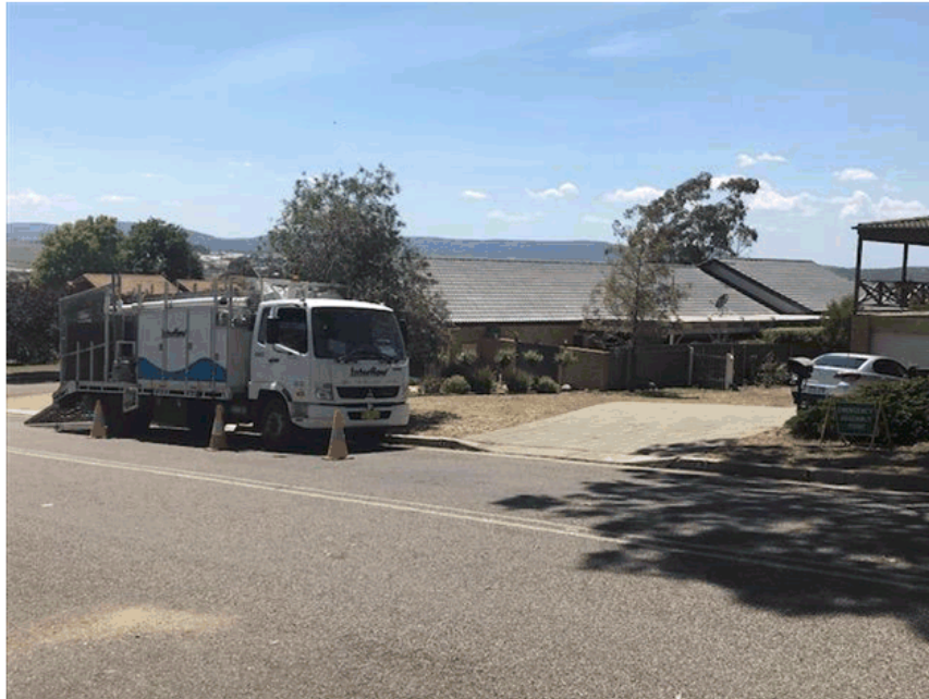
Interflow Relining crew
