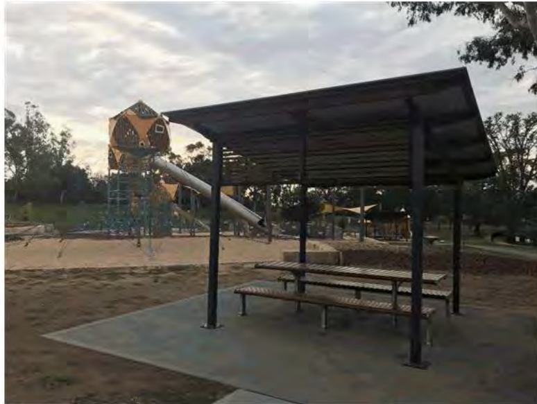
Example of shelter being constructed at Rage Cage.
