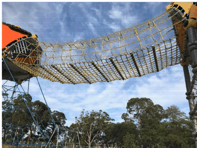
Completed repairs to Suspended Walkway at Adventure Playground.
