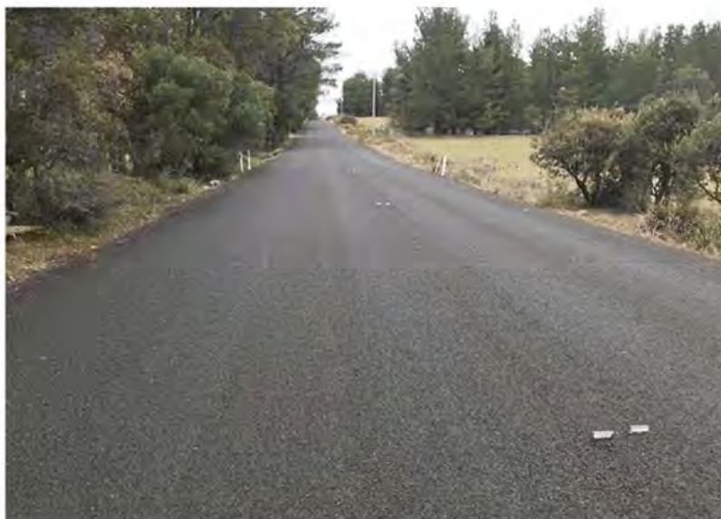
Highland Way Resealing
