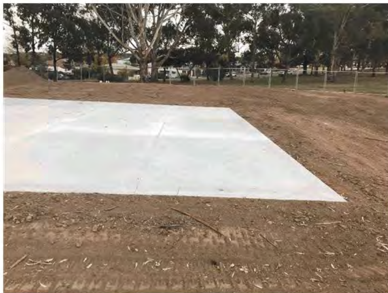
Commencement of mounds around the Rage Cage, looking towards Verner Street
