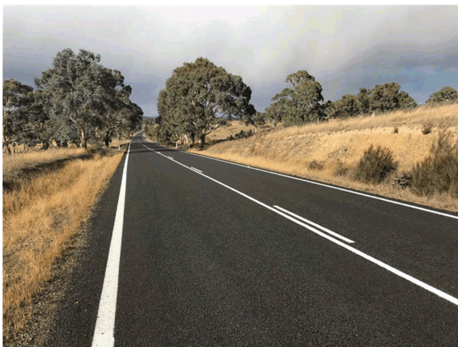
Bungendore Road – Heavy patching, reseal and line marking completed
