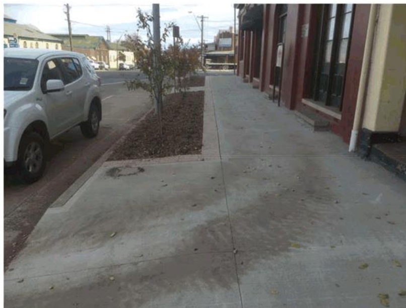
Concrete Works - Mandelsons
