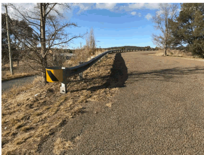
Guard rail repair - Old Sydney Road
