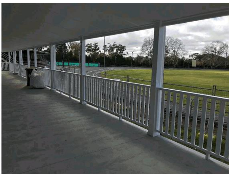
Seiffert Oval Pavilion – looking over onto playing surface
