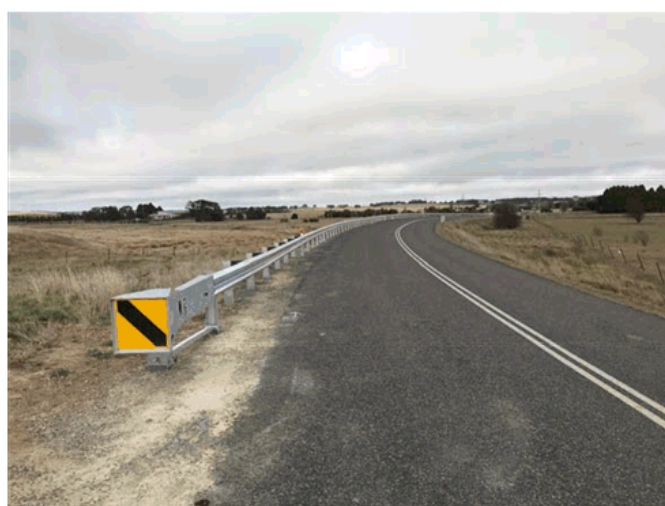
Guard rail repair – Fifes Bridge, Windellama Road
