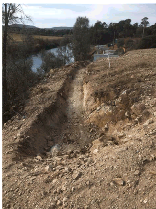
Approaches to bridge
