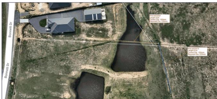
Photo: Pipe Burst Bonnett Drive Goulburn
