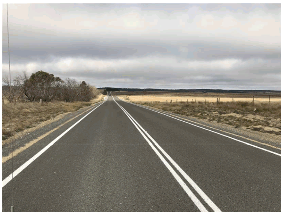
Windellama Road Widening – works completed
