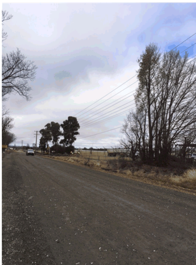
Bungonia Road – reconstructed sub base with gravel layer
