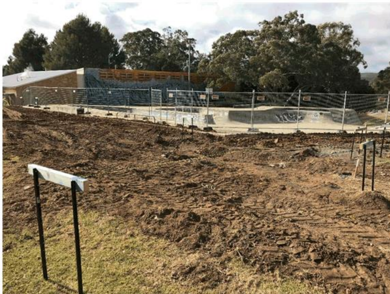
Skate Park – construction phase, Deccan Street frontage
