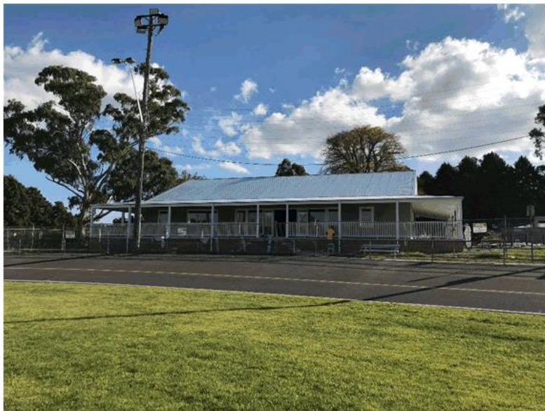
Seiffert Oval Pavilion – picket railing installation
