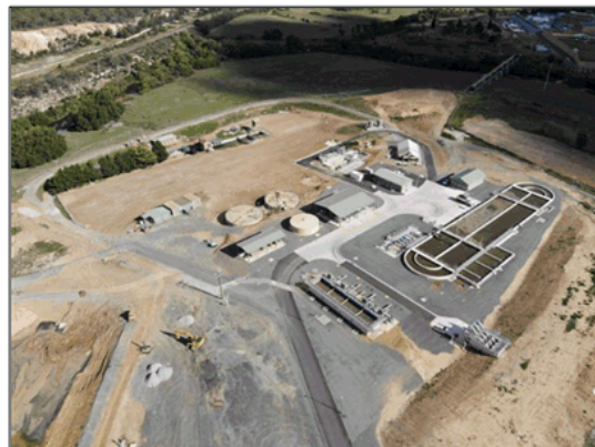
Photo: Goulburn Waste Water Treatment Plant
