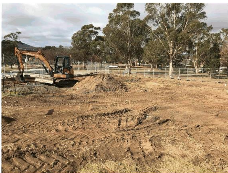
Skate Park – construction phase looking towards Adventure Playground
