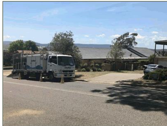
Photo: Interflow Relining Crew
