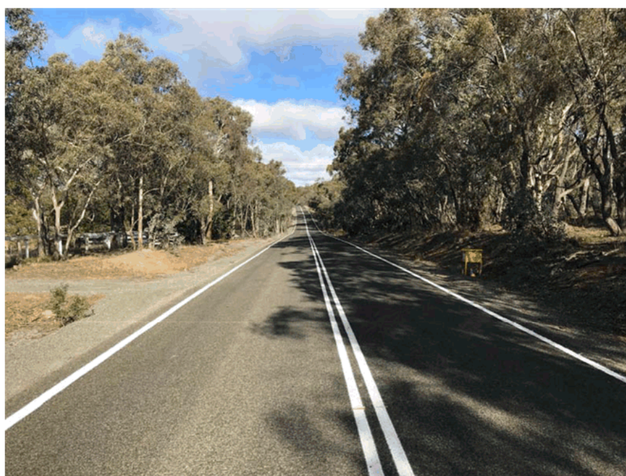
Range Road – Heavy patching, reseal and line marking completed
