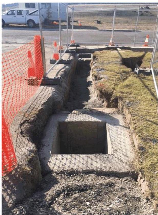
Racecourse Drive – stormwater pits and trench
