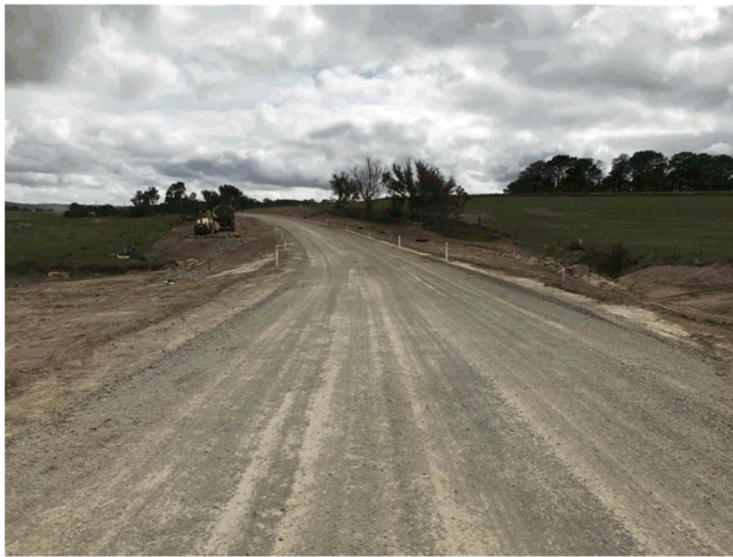
Curve re alignment on Pomeroy Road
