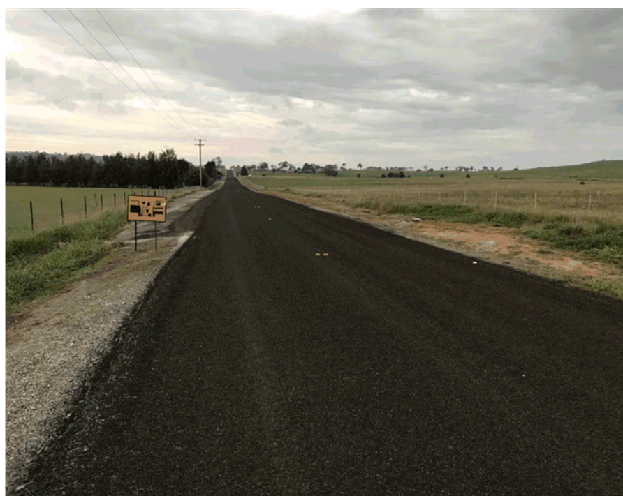
Middle Arm Road widening & bitumen over seal
