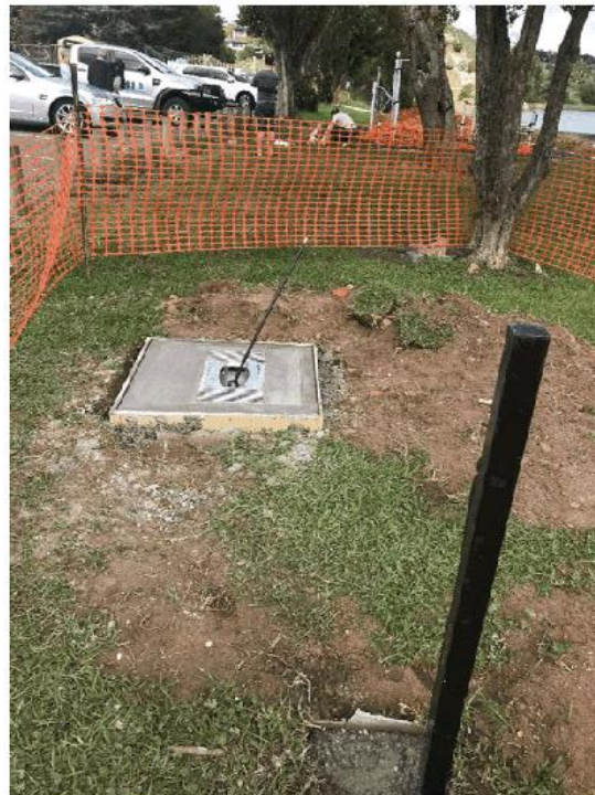
Marsden Weir Park Water Station
