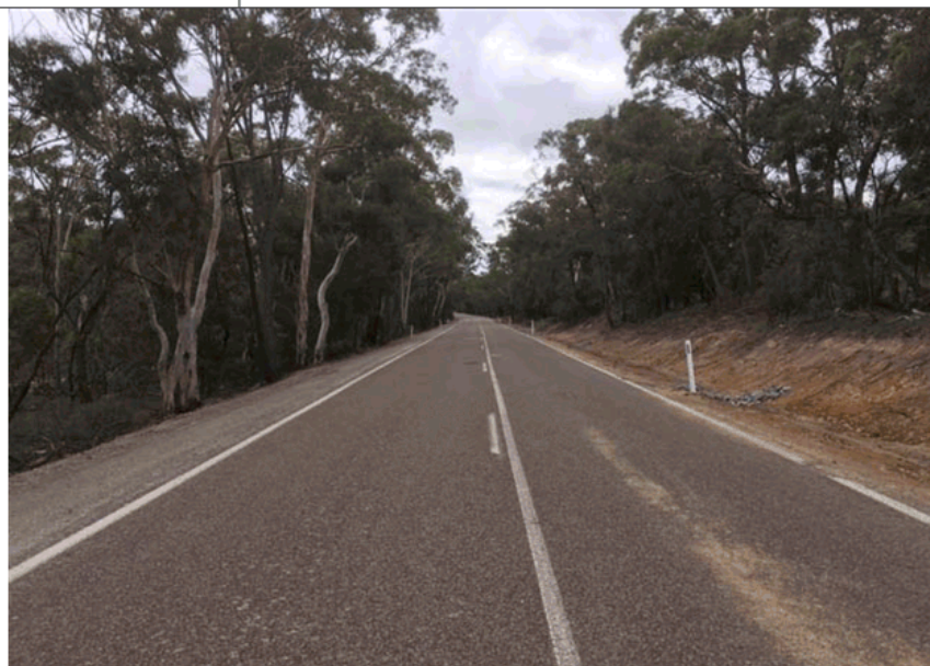
Taralga Road drainage & edge works
