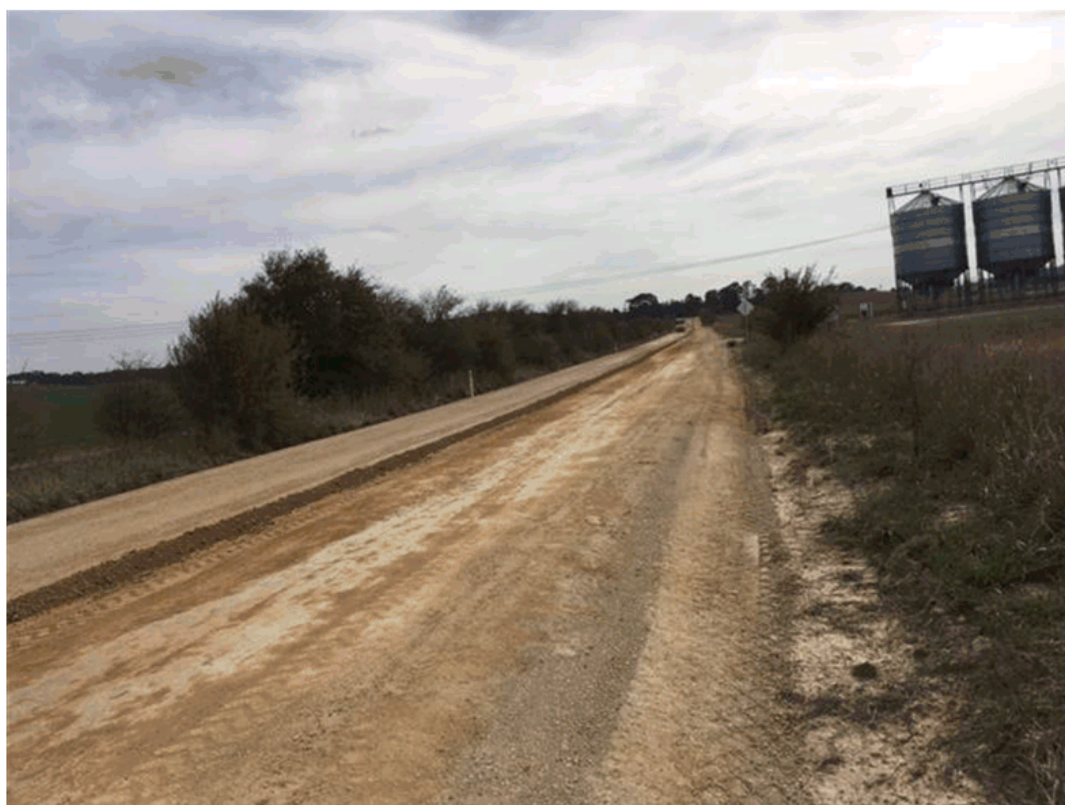
Currawang Road – Ripped and ready for gravel overlay
