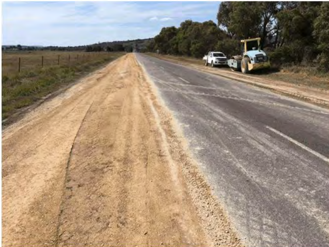
Windellama Road – Shoulder resheeting
