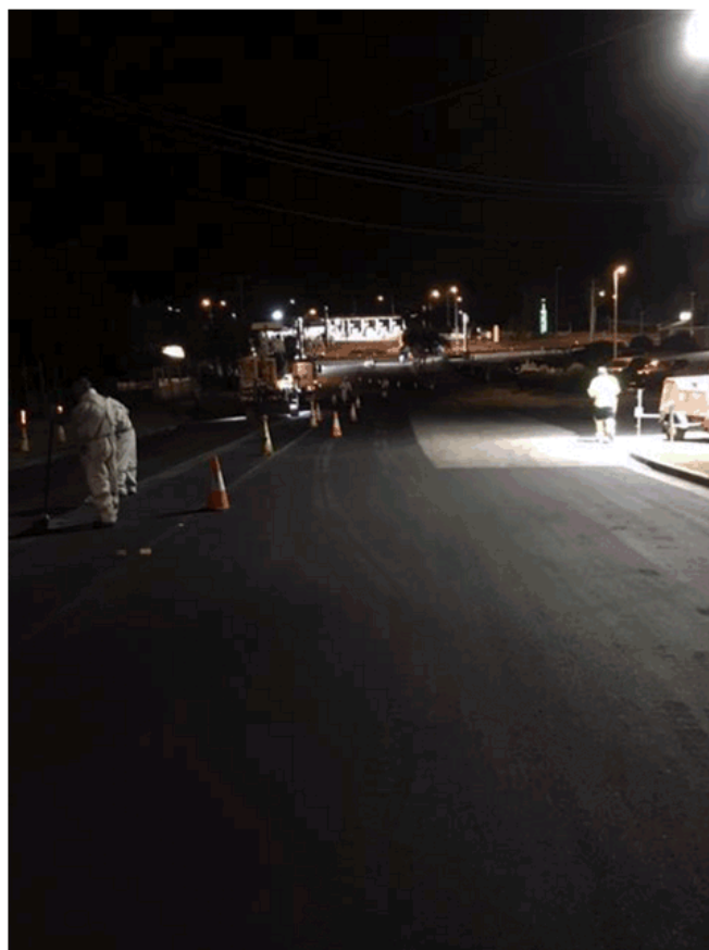
Sowerby Street – Asphalt Night Works
