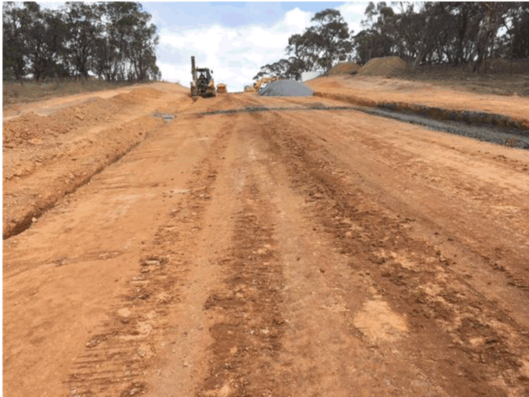
Mary Street Extension – Sub soil drain installation
