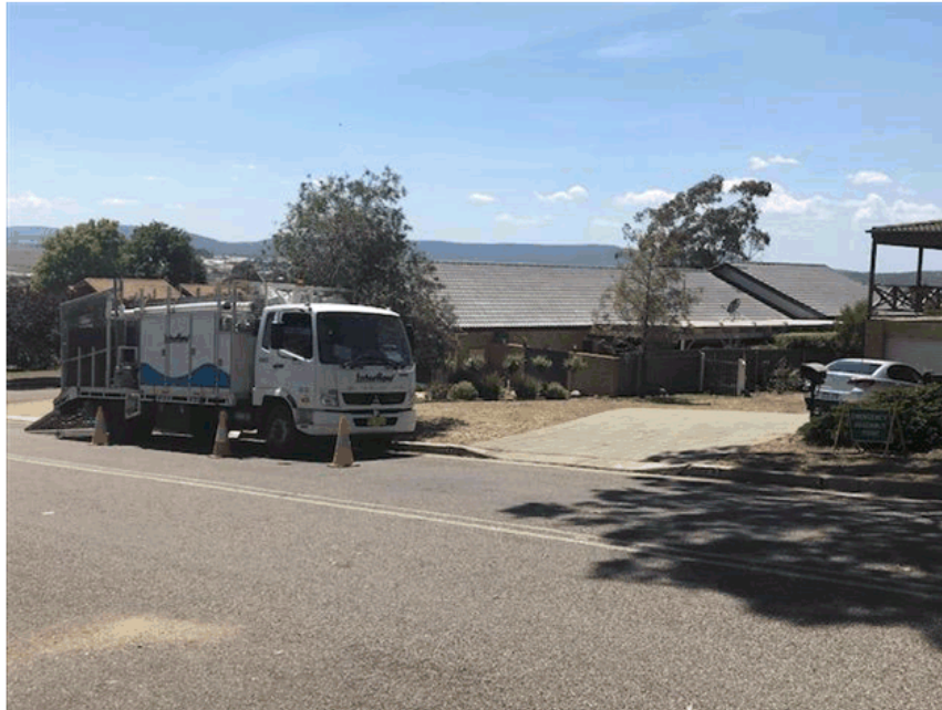
Interflow Relining crew
