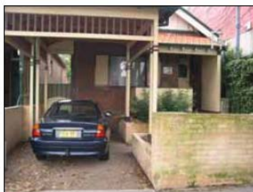
Intrusive carport which has removed a section of the original verandah and obscures the façade of the Federation cottage.
