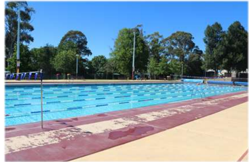
Stage 1 of the Goulburn Aquatic Centre (pictured above) is due to commence in 2019-2020
